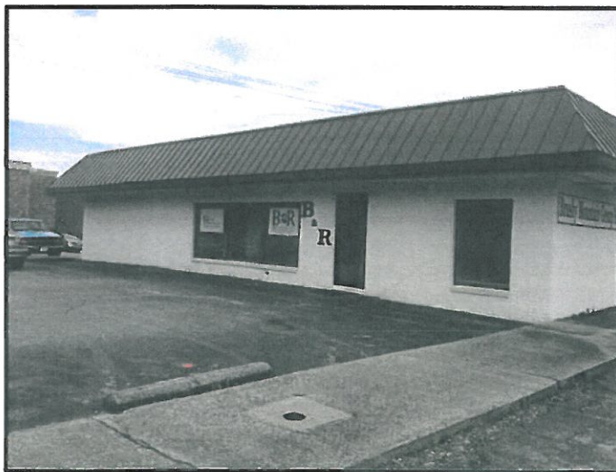
Existing B&R Building (Photograph Facing Approximately Southeast)
