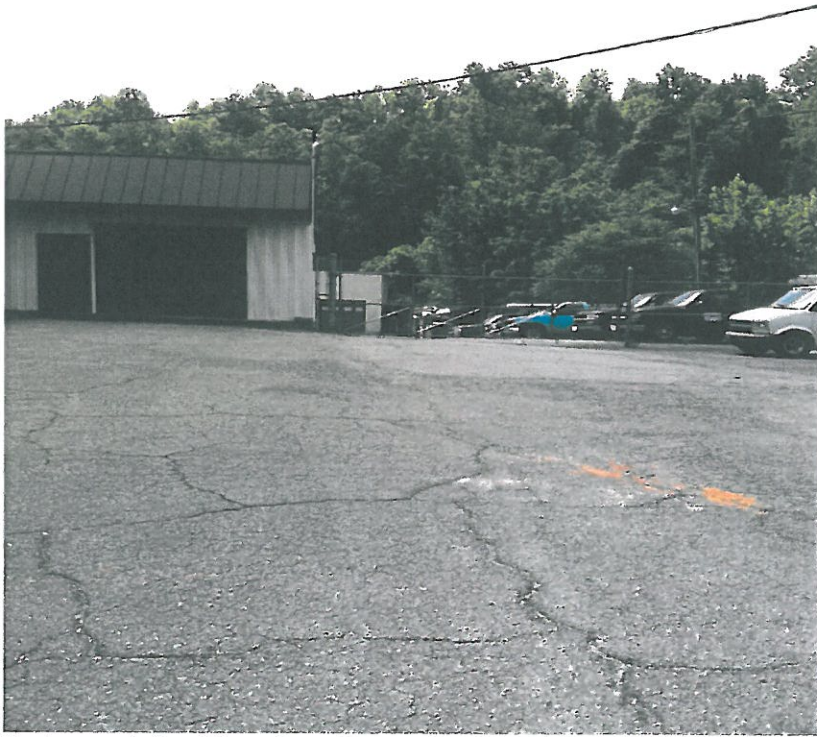
Photograph 3 – View from the north side of the site looking south.
