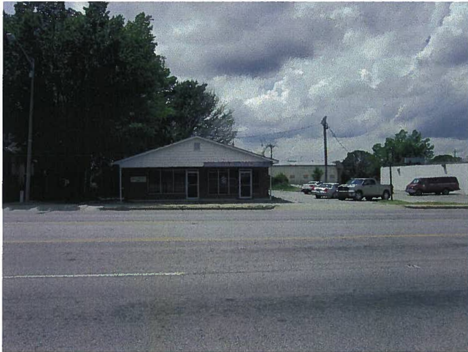
Parcel 197 (Ward Holdings LLC Property), looking west
