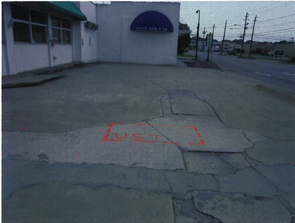
Parcel 105 (Vincent Peele Property LLC), looking west. Photo shows approximate marked location of probable UST No. 1 near the northeast corner of the parcel.
