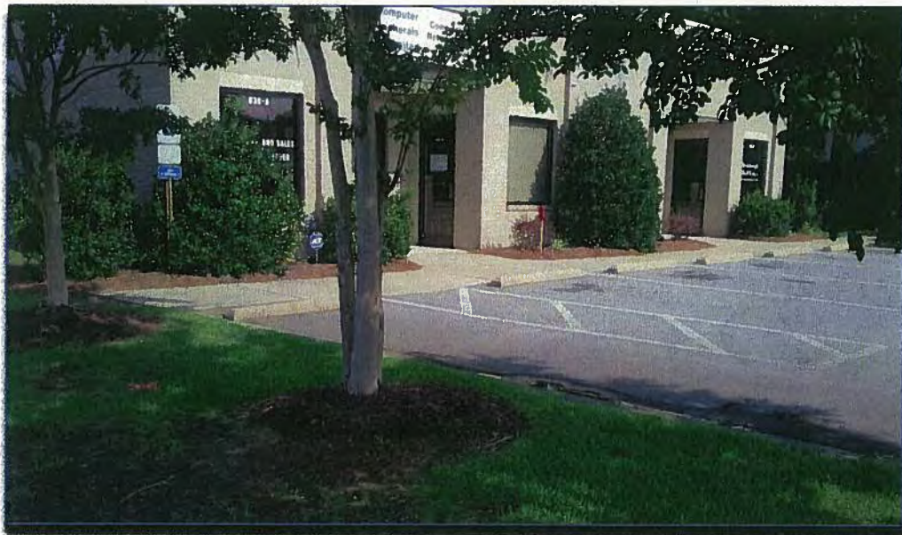
From South-central portion of property along West 10 th Street looking Northwest across site.
