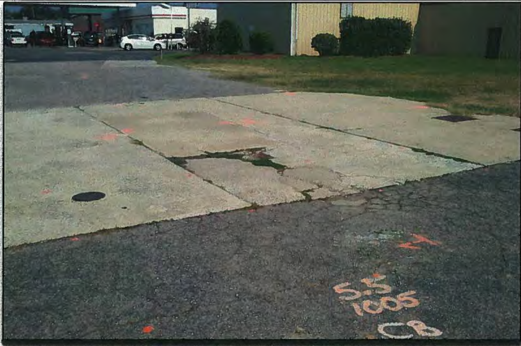
From near proposed catch basin 1005 (foreground) looking Northwest across the site.
