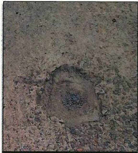
Former Western UST access port (assumed) filled with concrete.
