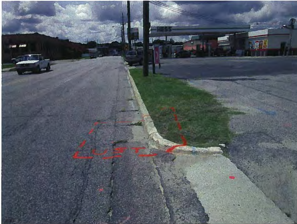
Parcel 101 (Walter L. Williams Property), looking west. Photo shows approximate marked location of probable UST No. 1 near the southwest corner of the parcel.
