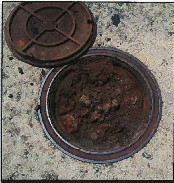
Former Eastern UST access manhole filled with concrete.
