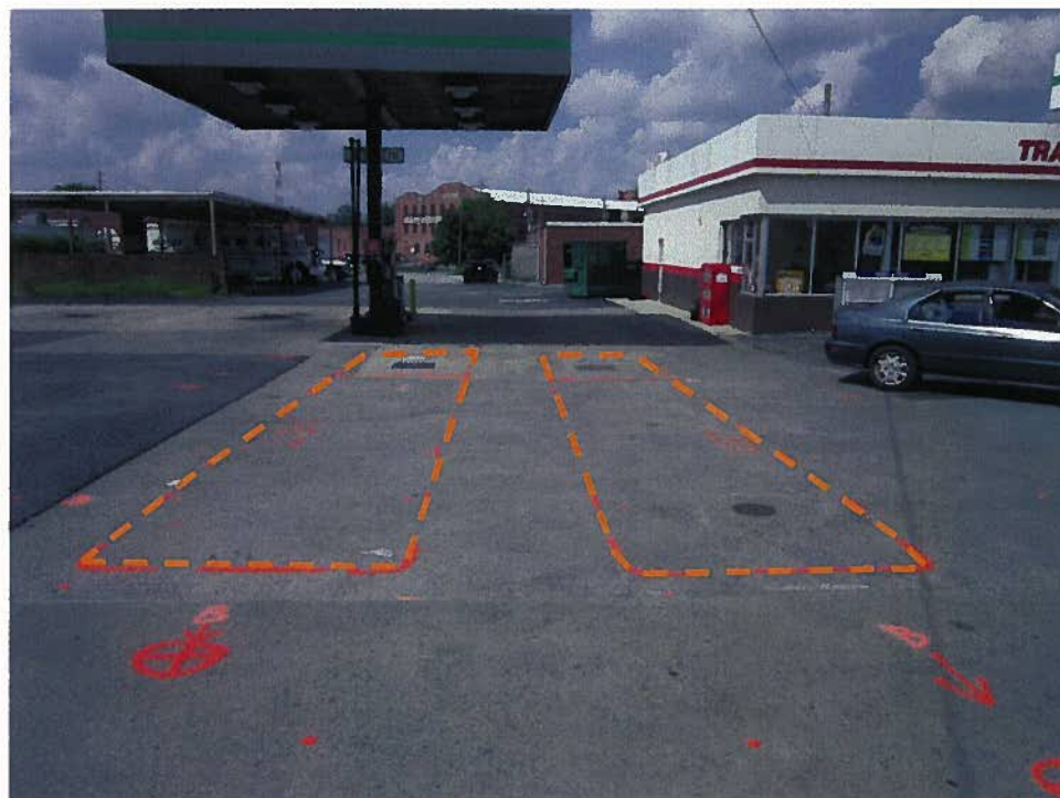
Parcels 97, 98, & 99 (Walter L. Williams Property), looking north. Photo shows approximate marked location of known UST Nos. 1 and 2 near the southwest corner of the westernmost building.
