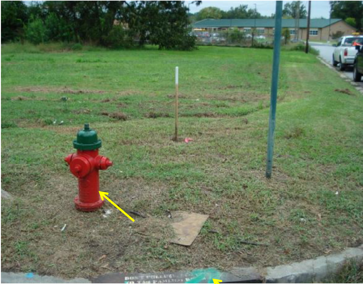
Fire Hydrant on corner of Pennsylvania and Myrtle. Storm at bottom of photo
