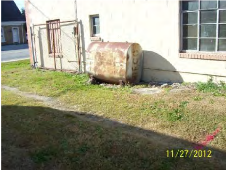
Picture shows AST on side of building
