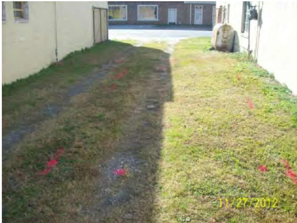
Picture shows Gas and Electric lines marked in pink
