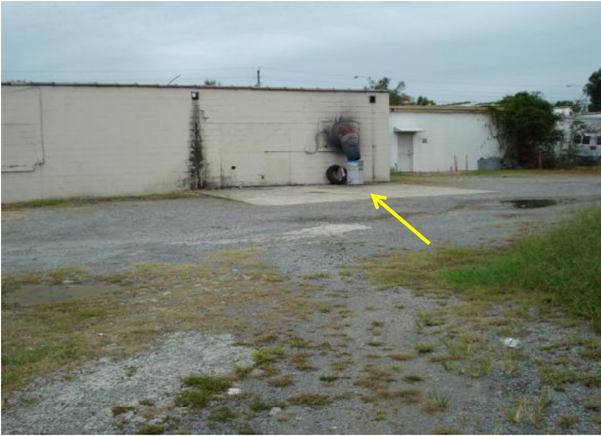
Concrete pad with rebar in concrete Target A
