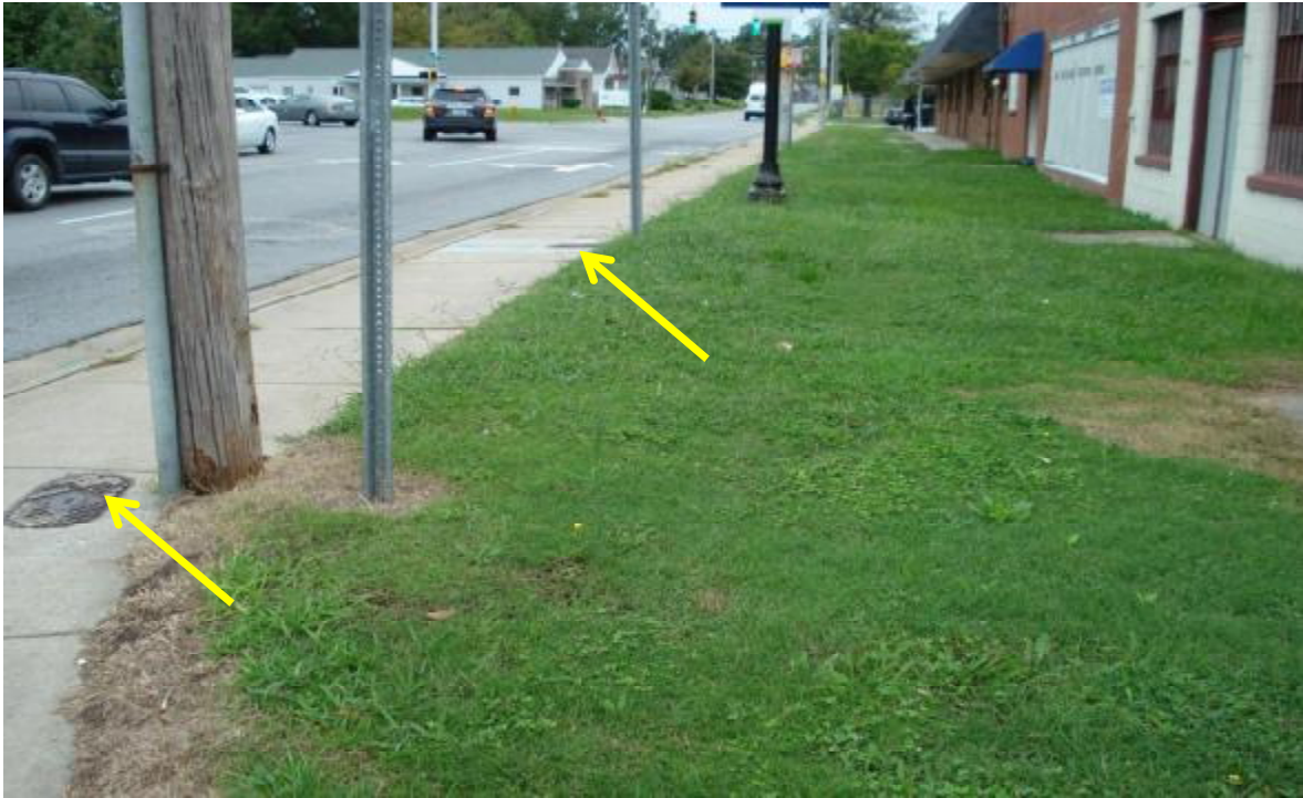
Traffic Control from pole to junction box and water meter with service to building along W 14th
