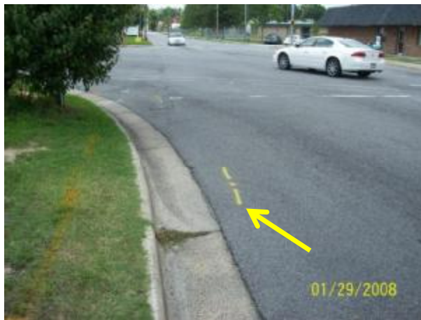
View of corner of property at W 14 th and Farmville Gas line delineated in yellow. Next to tree is NCDOT hand hole with fiber coming down pole.
