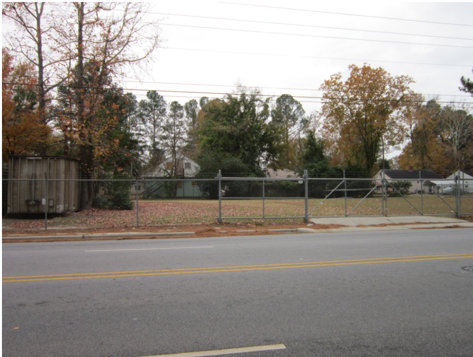
Parcel 18 (Phillip Ray Cox Property), looking south
