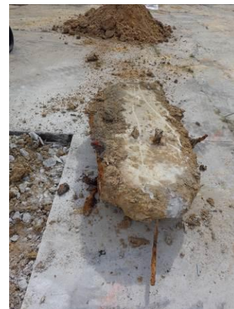
Photo #6 Concrete and Metallic Mass Initially Identified during GPR
