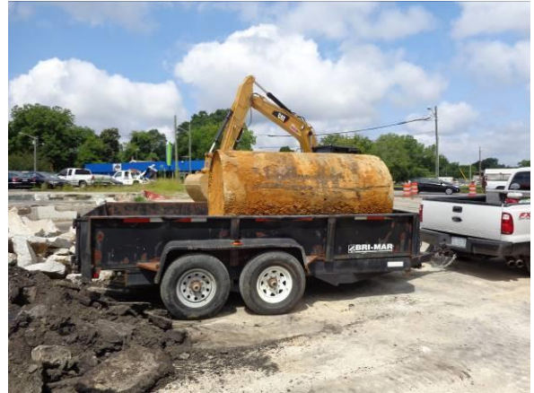
Photo #14 UST Removed and Loaded onto Trailer for Disposal
