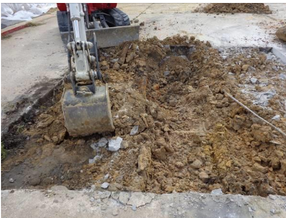
Photo #5 Initial Excavation at Western Potential UST Location
