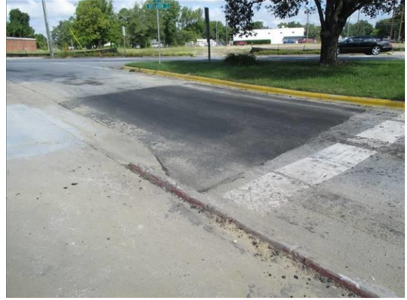
Photo #18 Asphalt Replaced on W 10 th St.
