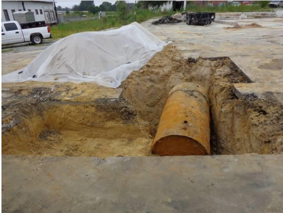
Photo #13 UST in Preparation for Removal
