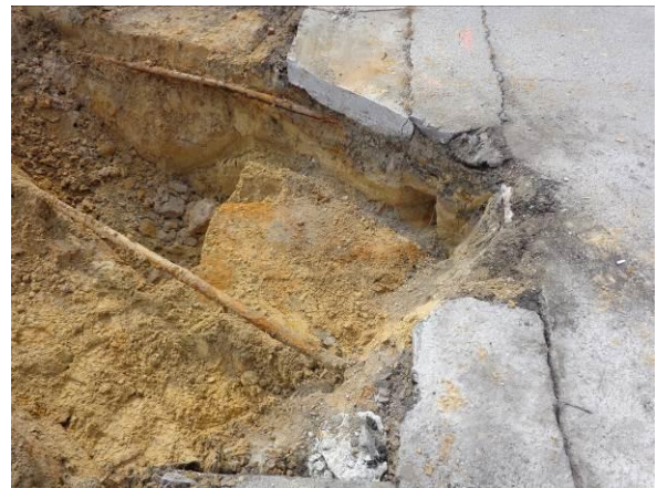
Photo #10 Initial Excavation and UST Discovery (Eastern Location)
