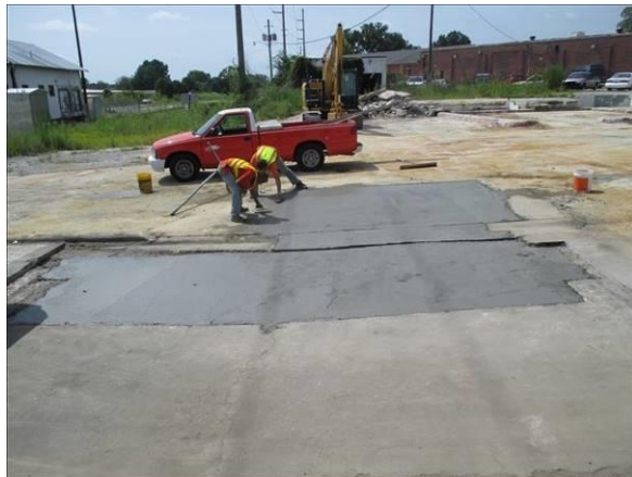
Photo #17 Surface Concrete Replaced
