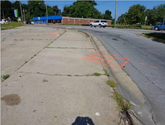
Photo #1 View of Parcel 186 Facing Northwest
