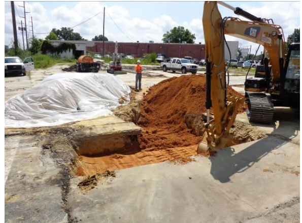
Photo #16 Excavation Backfilled with Imported Granular Soil
