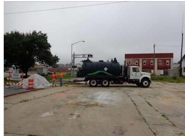
Photo #12 Vacuum Truck used to Empty Tank of Residual Fluids
