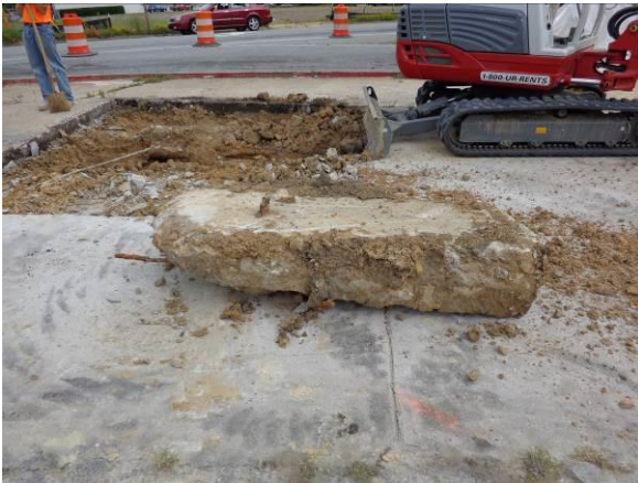
Photo #7 Concrete and Metallic Mass at Western Potential UST Location
