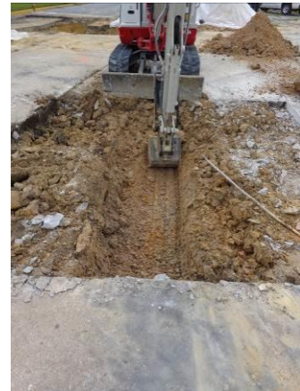
Photo #8 Excavation Extended Downward to Confirm Absence of UST
