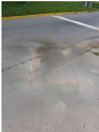
Photo #9 Concrete Cut at Eastern Potential UST Location
