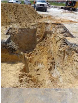
Photo #15 Empty Excavation after UST Removal
