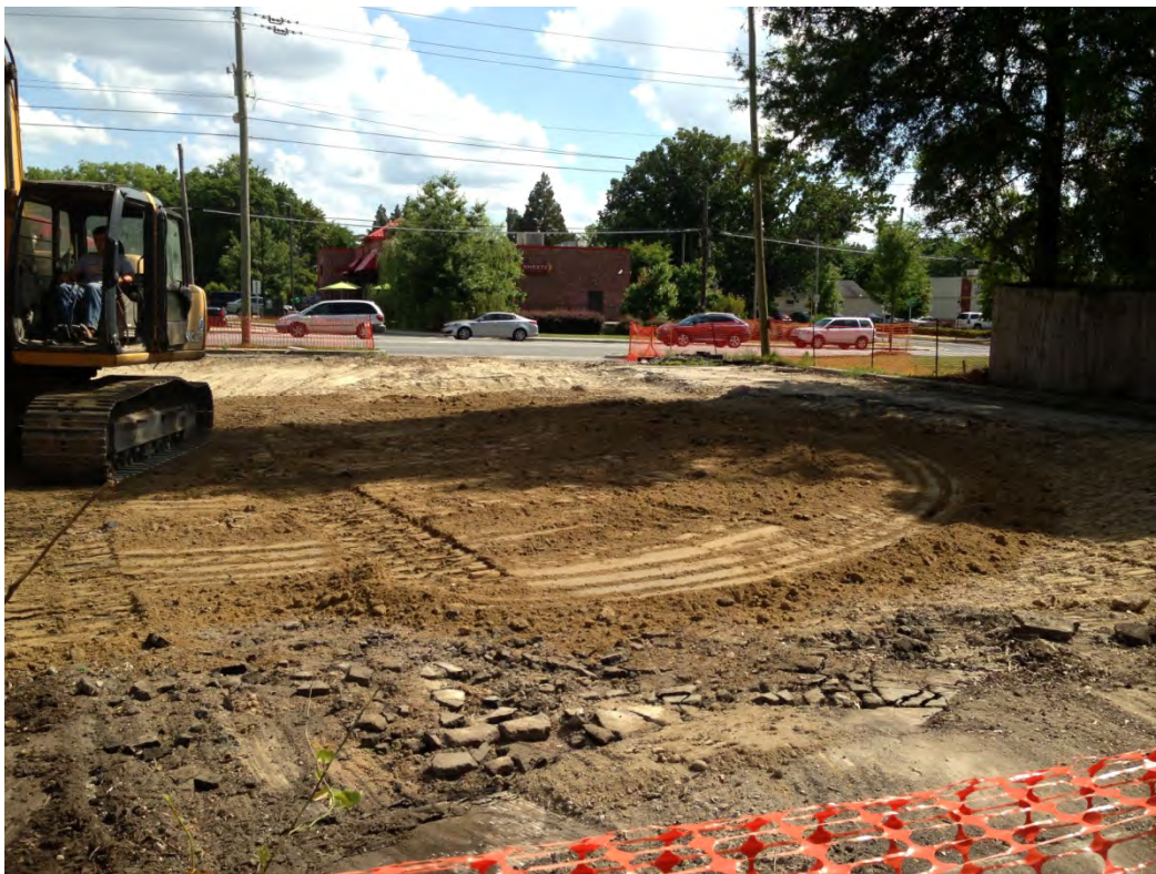
Photograph 8: View of the backfilled excavation. View is to the South.
