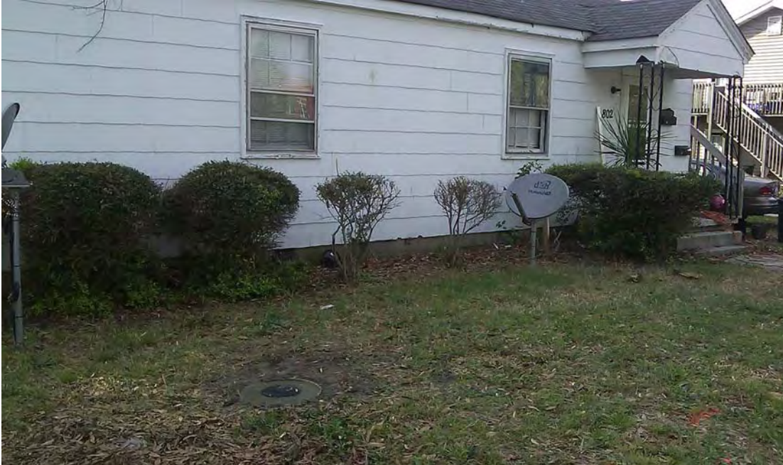
Photo 3. Looking northwest at MW-11 located at 802 Forbes Street
