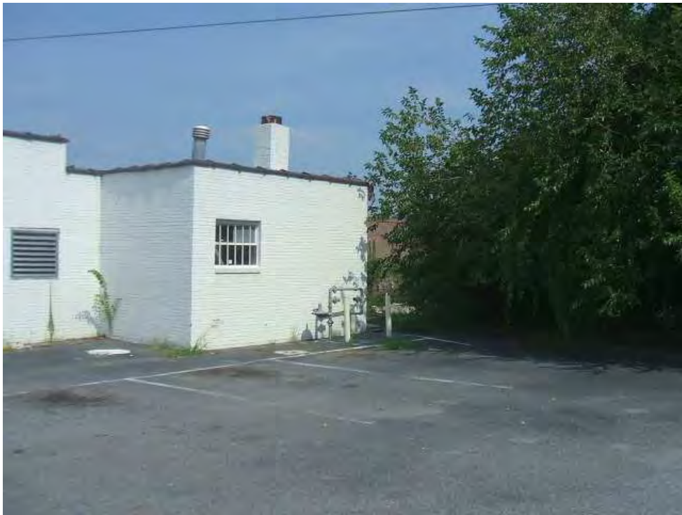
A view of the Northeast corner of the former dry cleaning facility. A monitoring well is located in the center of the picture, between the parking space and building.
