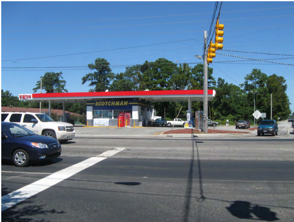
Parcel 48 (RI CS5, LLC Property), looking north
