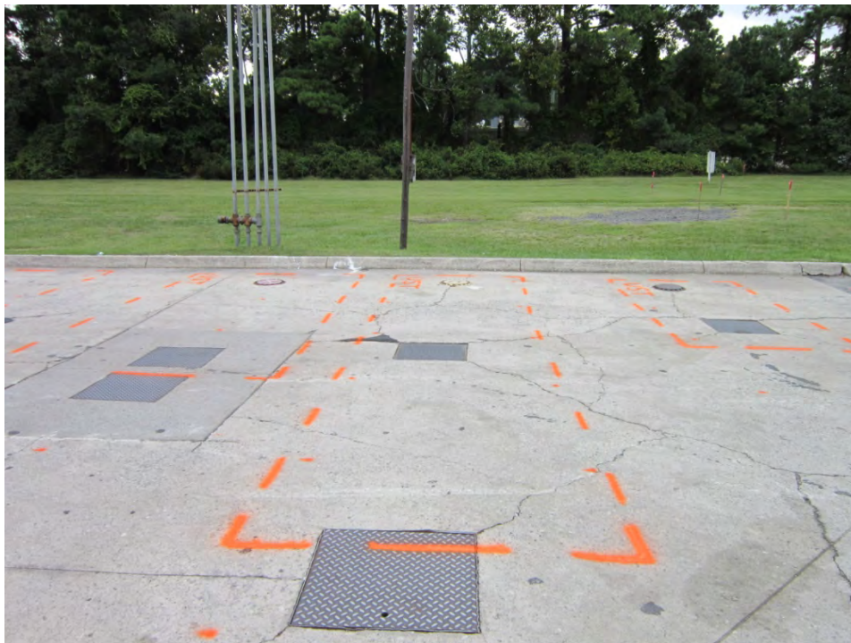
Parcel 48 (RI CS5, LLC Property), looking north. Photo shows approximate marked location of known UST Nos. 3, 4, and 5 near the northeast corner of the building.
