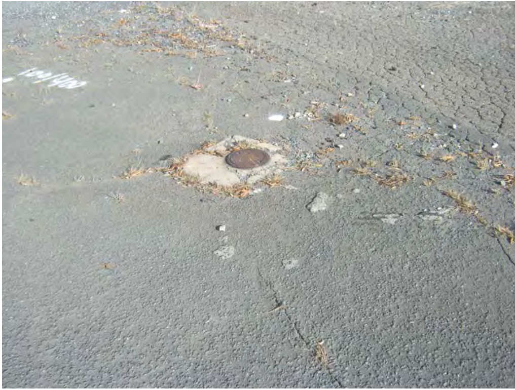
Photo 3 View of on-site groundwater monitoring well.
