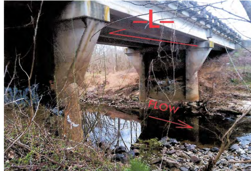
Profile of Bridge Looking Downstation from End Bent 2
