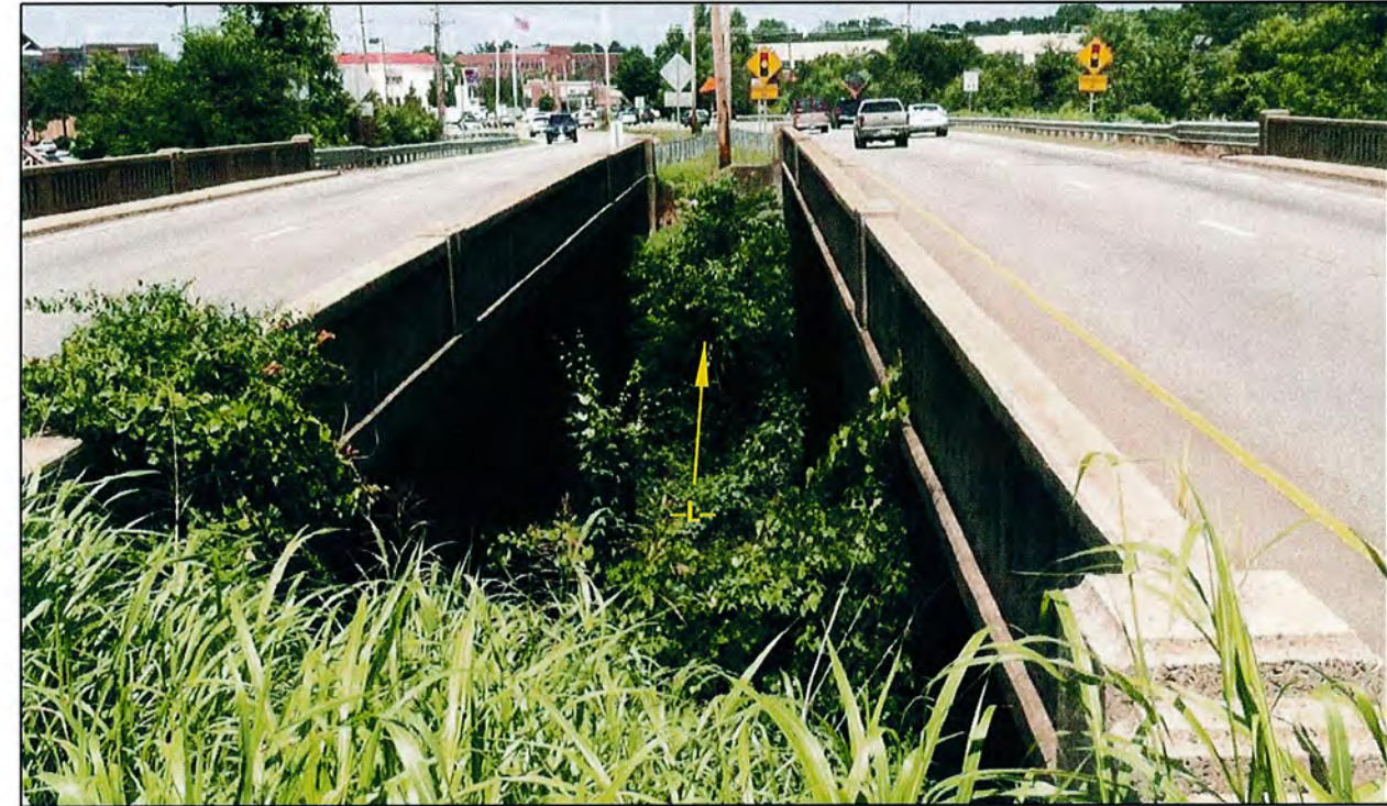
LOOKING UPSTATION ALONG -L- FROM NEAR EXISTING END BENT 1
