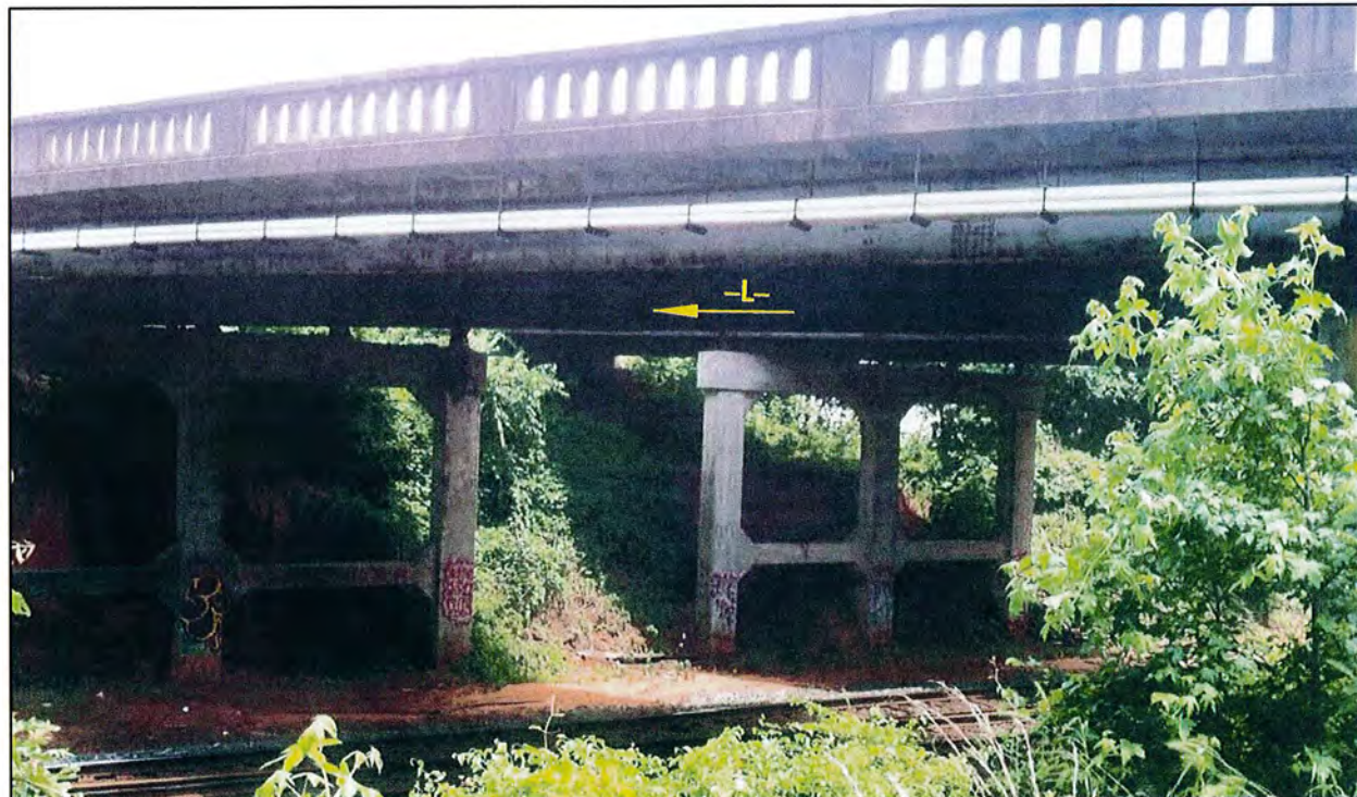
LOOKING SOUTH TOWARDS EXISTING BRIDGE FROM NEAR BORING DET-1
