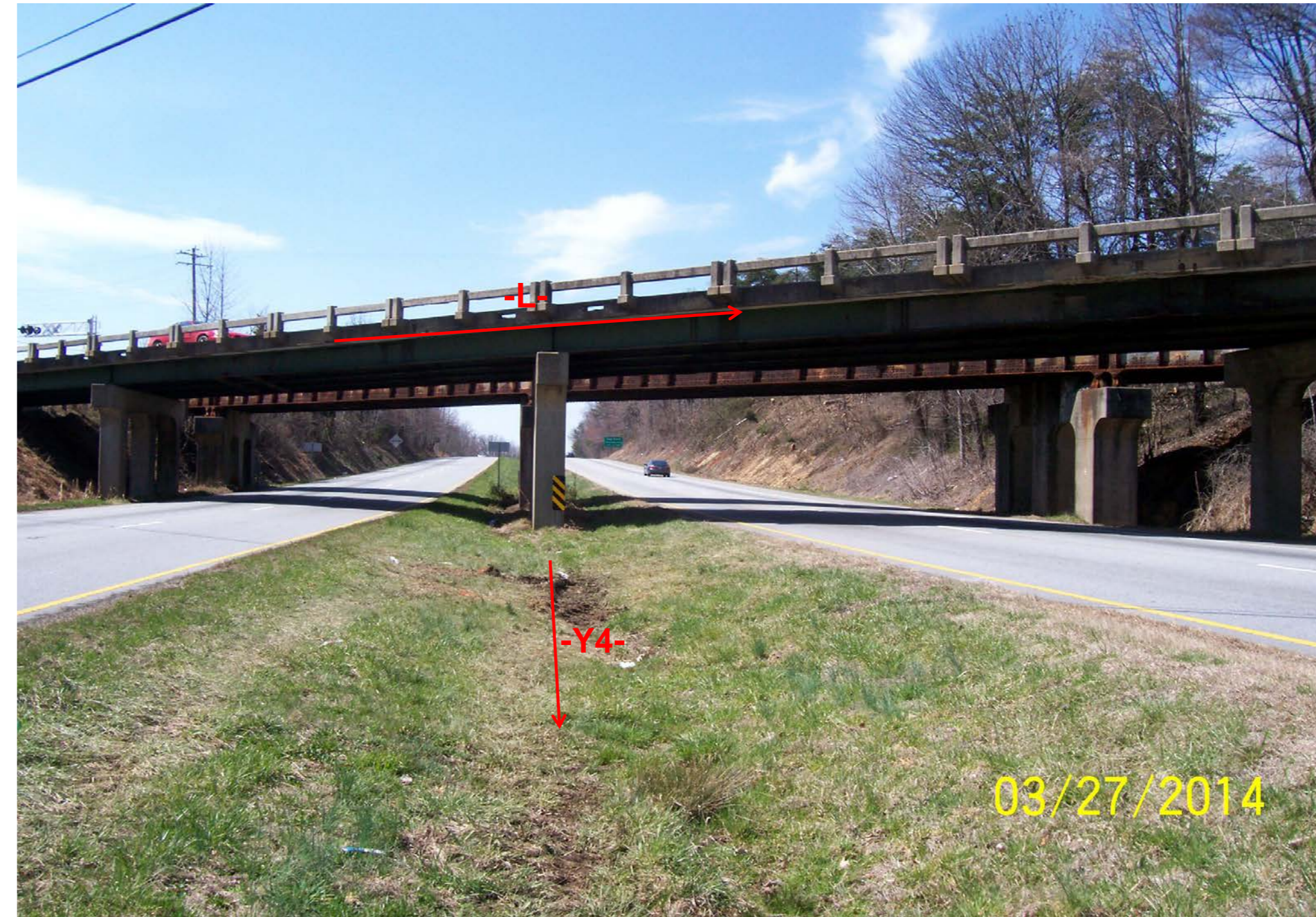
Profile of Bridge From B1-B Looking West
