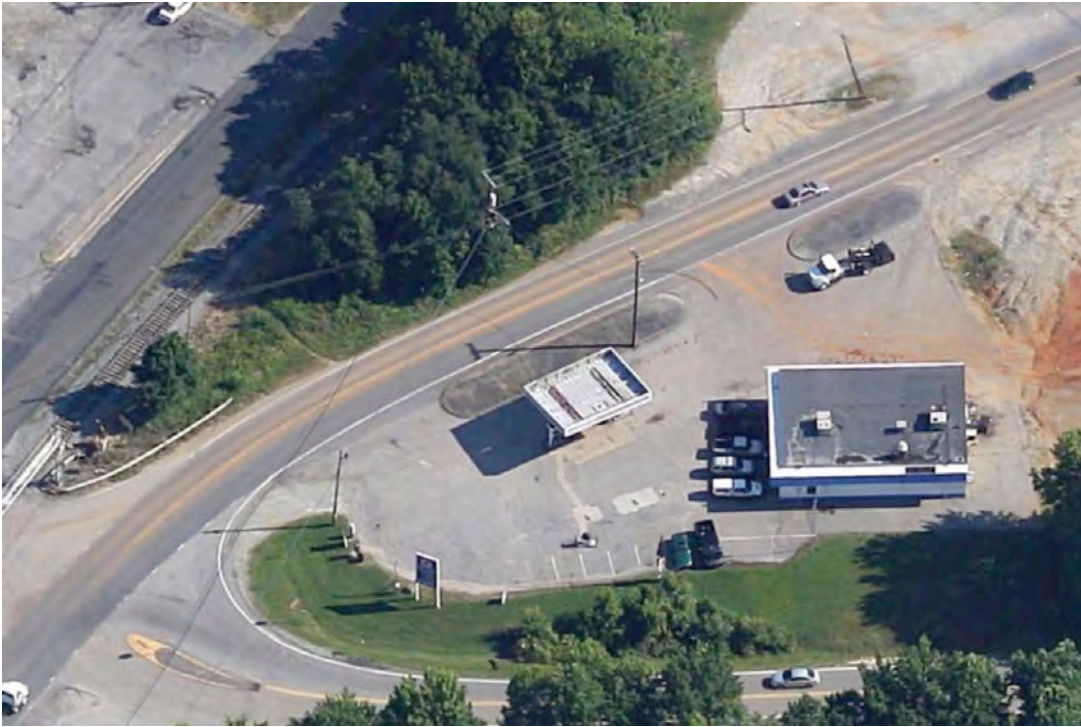
Photograph 1 : Oblique aerial view of 1611 Prospect Street. North is at top of photo (from Google Maps, 2014 imagery).
