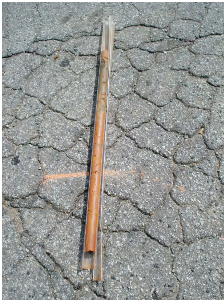
Photograph 7 : Photograph of core extracted from center of unidentified EM-61 anomaly.
