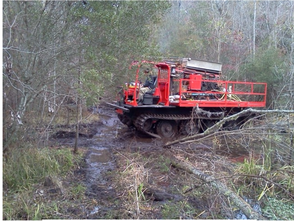
END BENT TWO FACING SOUTH ALONG -L- CENTER LINE
