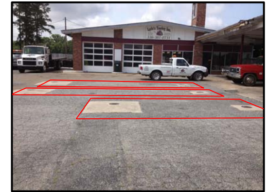
Approximate locations of 3 former gasoline/diesel known USTs
