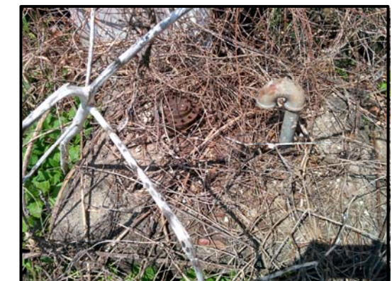
Vent pipe observed at location of probable kerosene/waste oil UST
