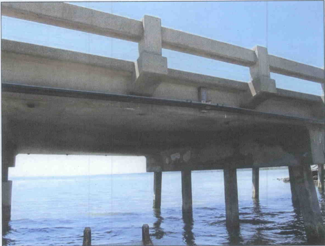
SPAN 6 UNDERSIDE. SIMILAR IN ALL SPANS.
