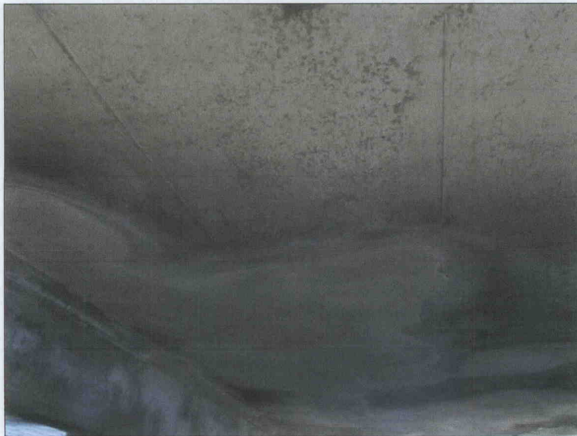
SPAN 32 DECK UNDERSIDE REPAIRED SINCE THE LAST INSPECTION.
