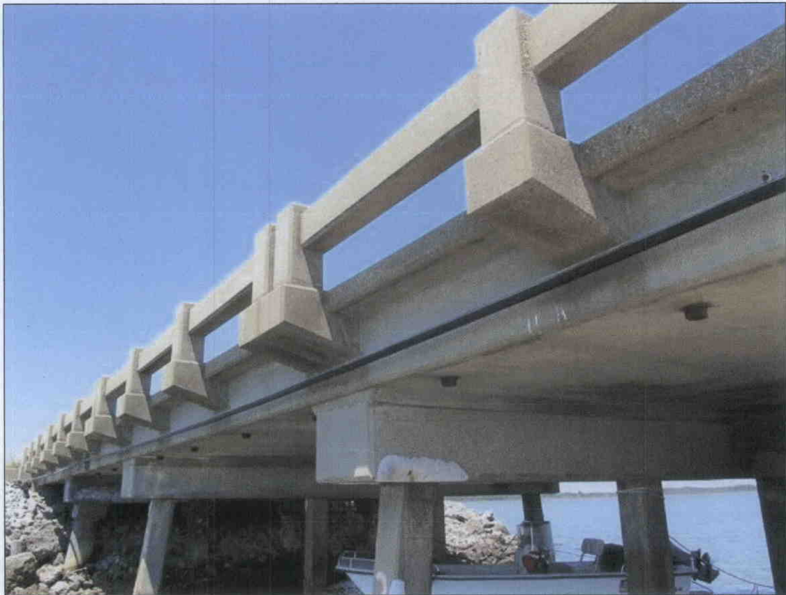
CABLE UTILITY ALONG THE SOUTH SIDE.
