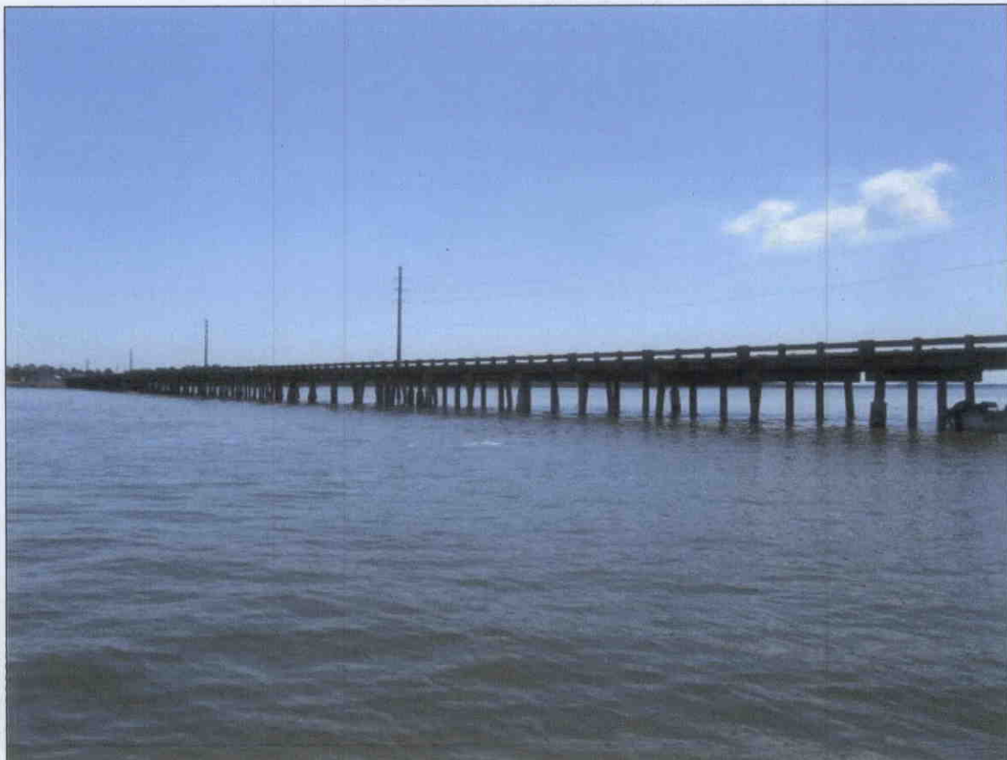
NORTH SIDE, LOOKING EAST.
