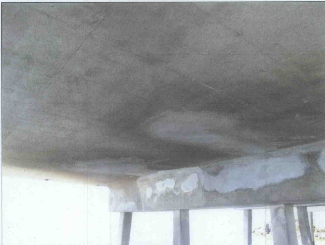
SPAN 6 DECK UNDERSIDE REPAIRED SINCE LAST INSPECTION.
