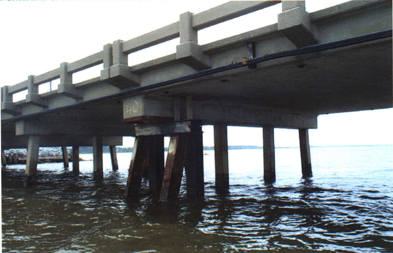
SPAN 40 SIDE OF BENT 40 W/ STEEL CRUTCHBENT (STEEL CRUTCHBENT @ ORIGINAL PILE 1)
