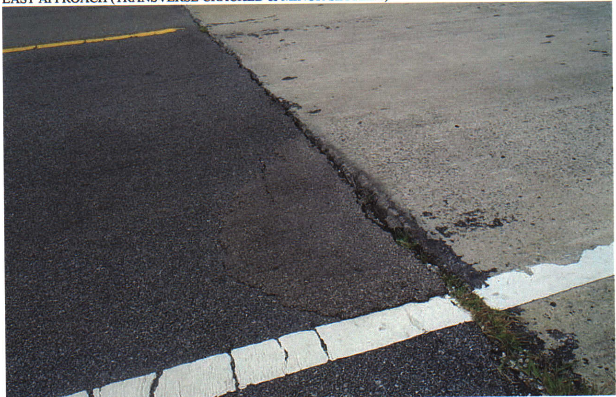
EAST APPROACH (MINOR SETTLED @ THE W.B.L.)
