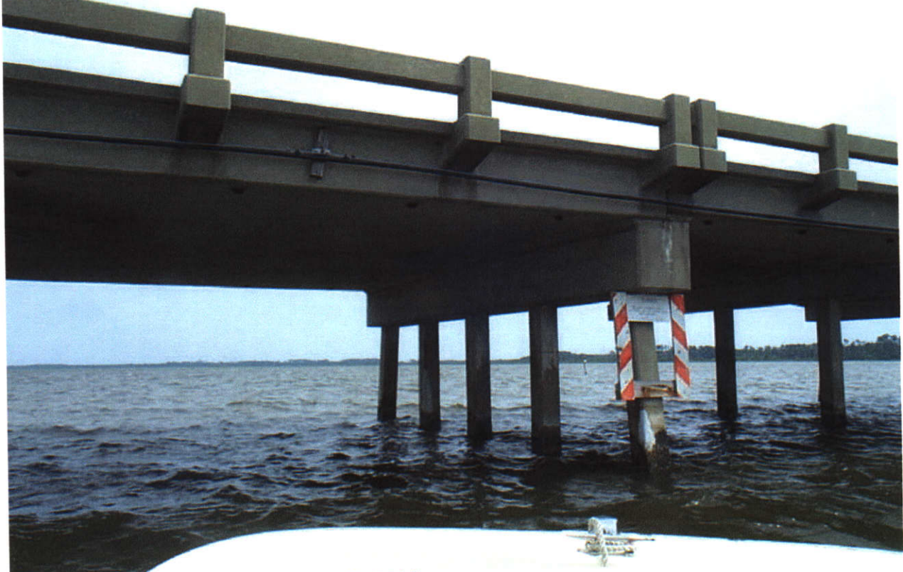
SPAN 24 SIDE OF BENT 24 (CHANNEL SPAN 24)
