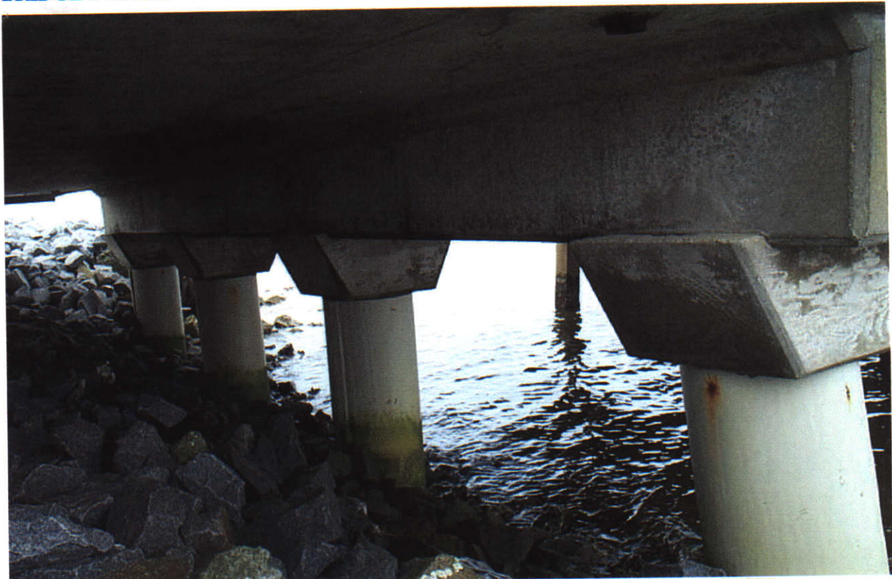
SPAN 47 SIDE OF BENT 46 (PILES 1- 4 ENCASED, SIMILAR BENT 1 & PILES 1- 4 ENCASED)
