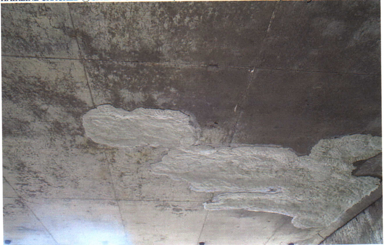
REPAIRS @ THE UNDERSIDE OF SPAN 28
