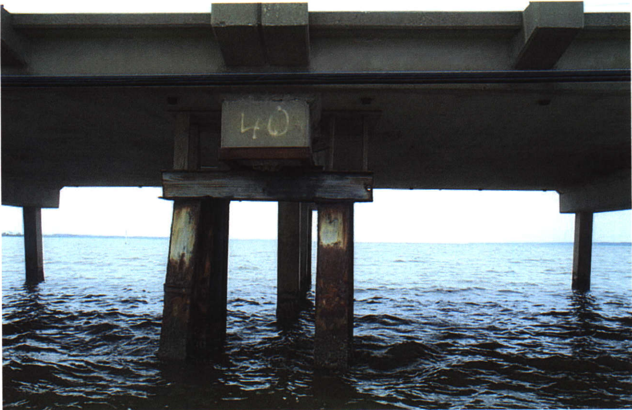
NORTH END OF BENT 40 W/ STEEL CRUTCHBENT
