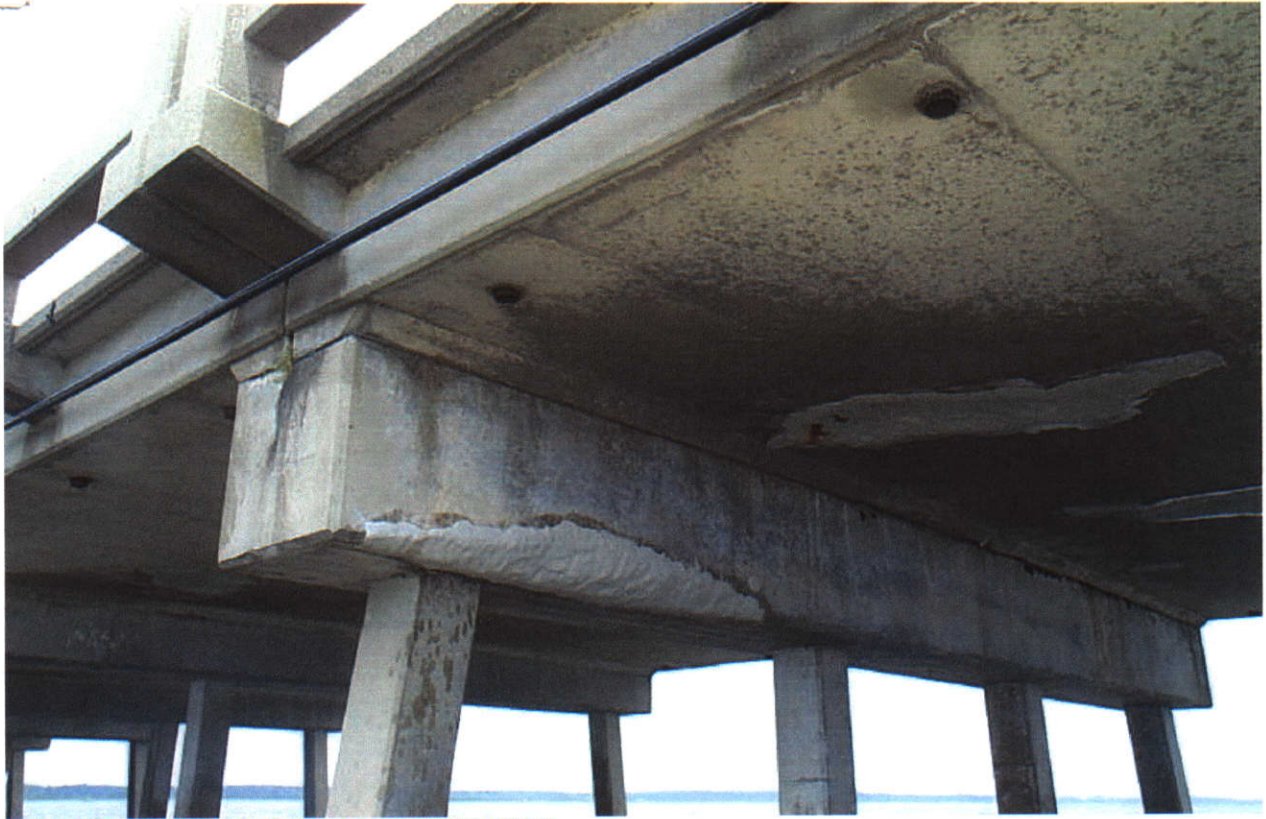
REPAIRS @ BENT 32 & SPAN 33 UNDERSIDE
