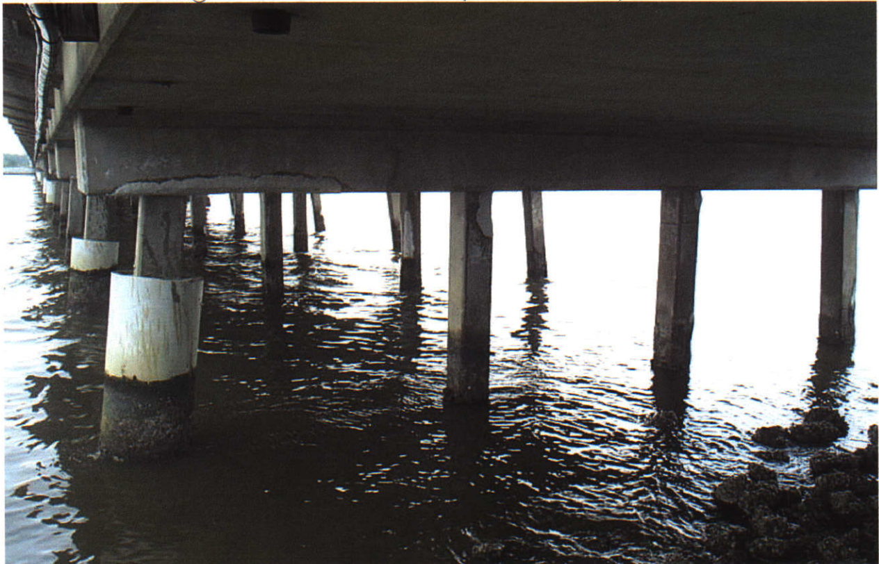
CAP & PILE REPAIRS @ SPAN 2 SIDE OF BENT 2
