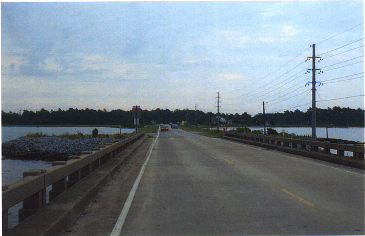
LOOKING EAST OFF BRIDGE
