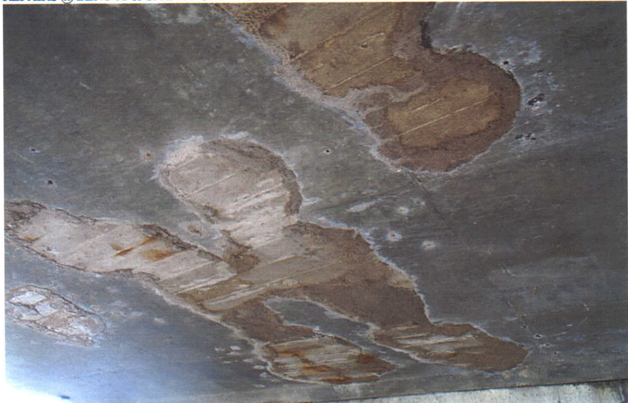
REPAIRS @ SPAN 43 UNDERSIDE
