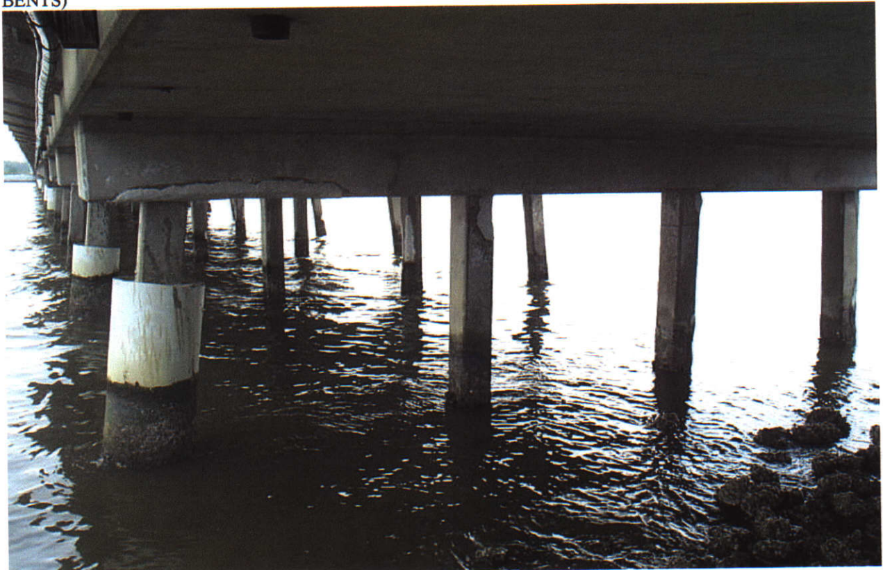
SPAN 2 SIDE OF BENT 2 (PILE 1 ENCASED)
