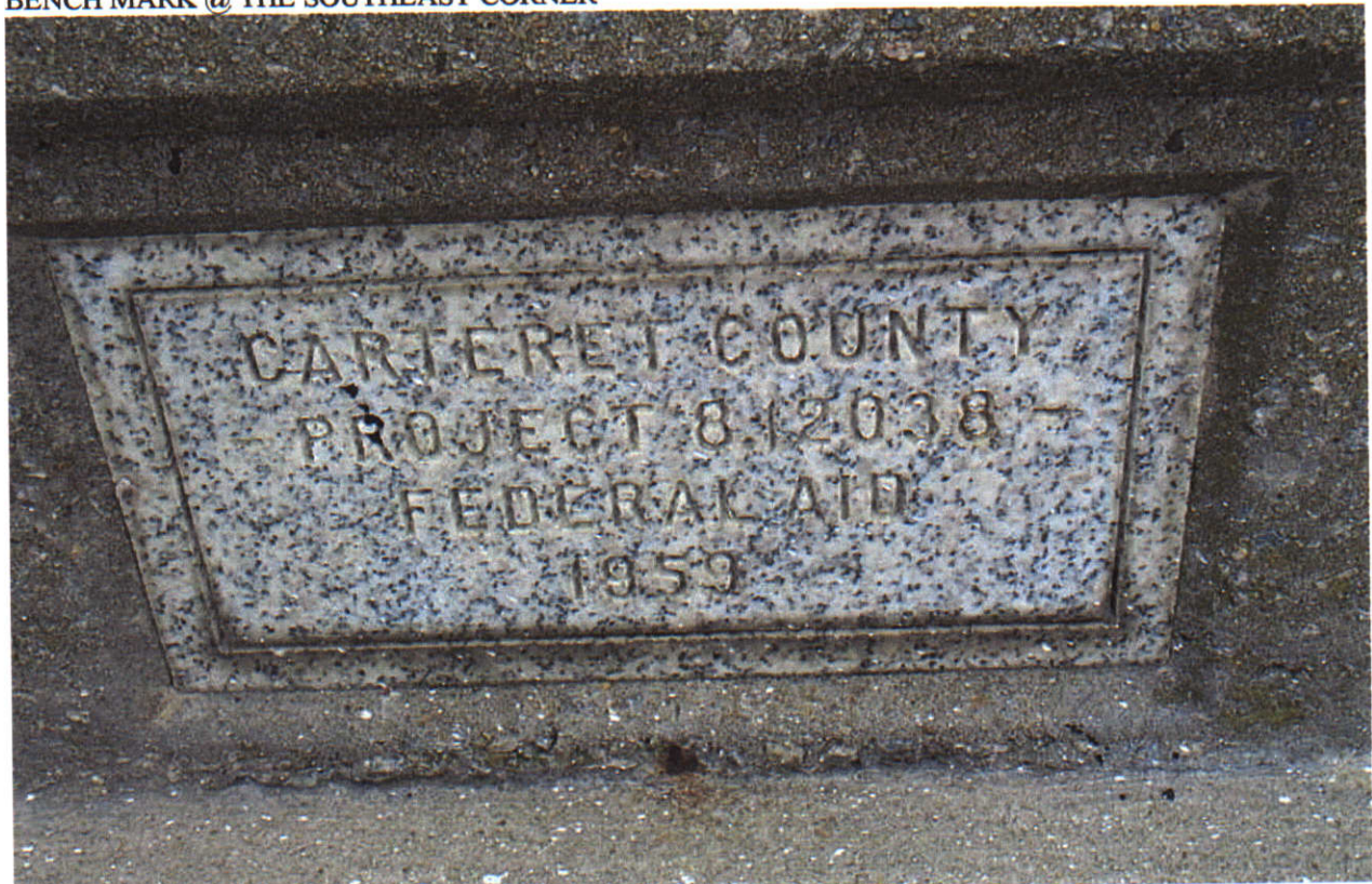
DATA PLATE @ THE NORTHEAST CORNER
