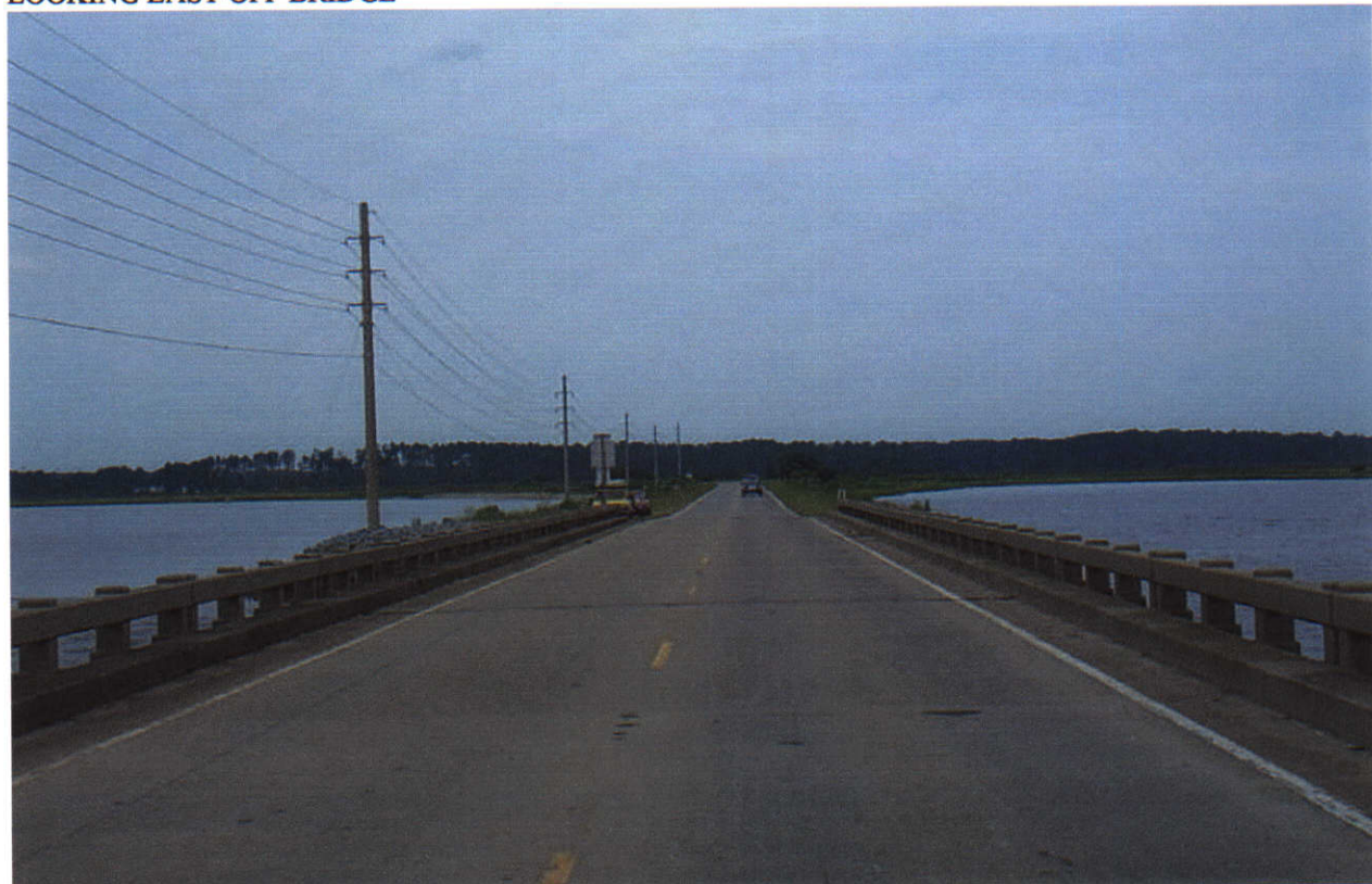
LOOKING WEST OFF BRIDGE
