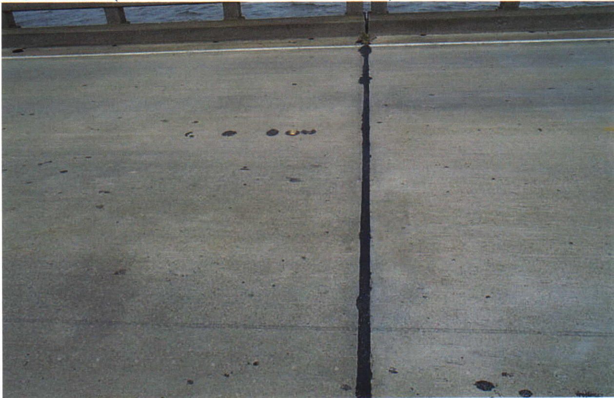
BENT 5 JOINT (SEALED)
