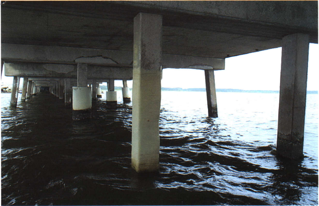
REPAIR ON PILE 3 @ SPAN 13, BENT 12
