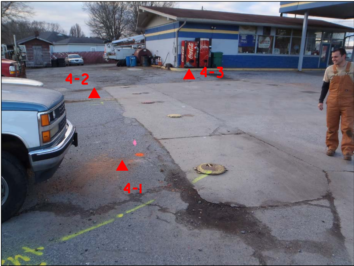
PHOTO 1 - BORINGS AT EXISTING UST BASIN LOOKING NORTHWEST
