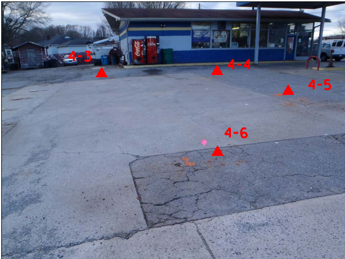
PHOTO 6 - BORINGS AT EXISTING UST BASIN LOOKING WEST
