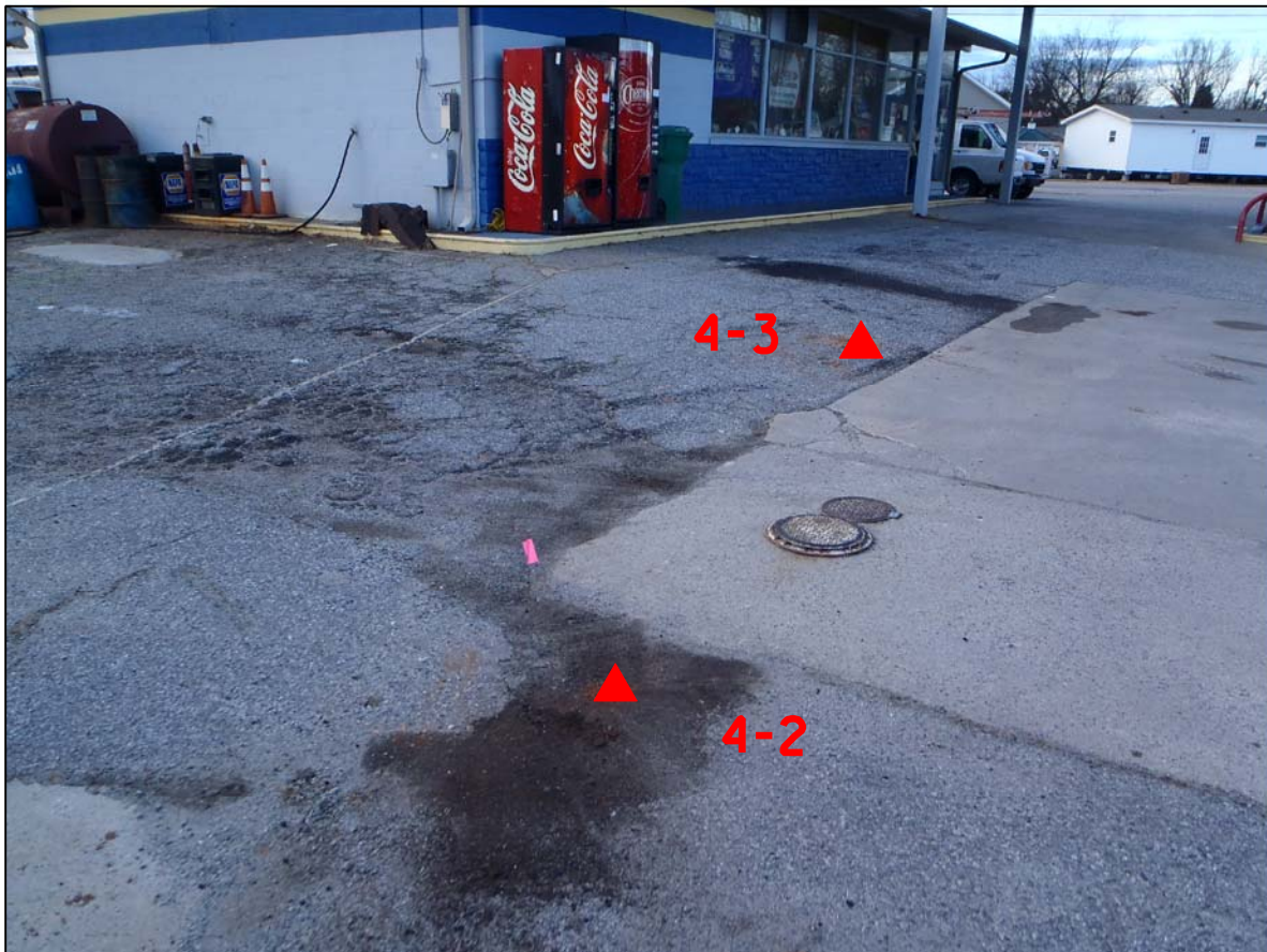
PHOTO 2 - BORINGS AT EXISTING UST BASIN LOOKING NORTH
