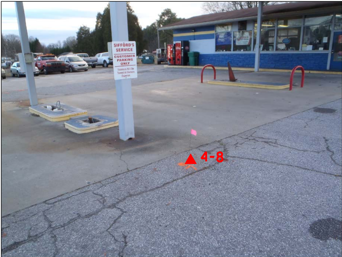
PHOTO 7 - BORING AT FORMER PUMP ISLAND LOOKING SW
