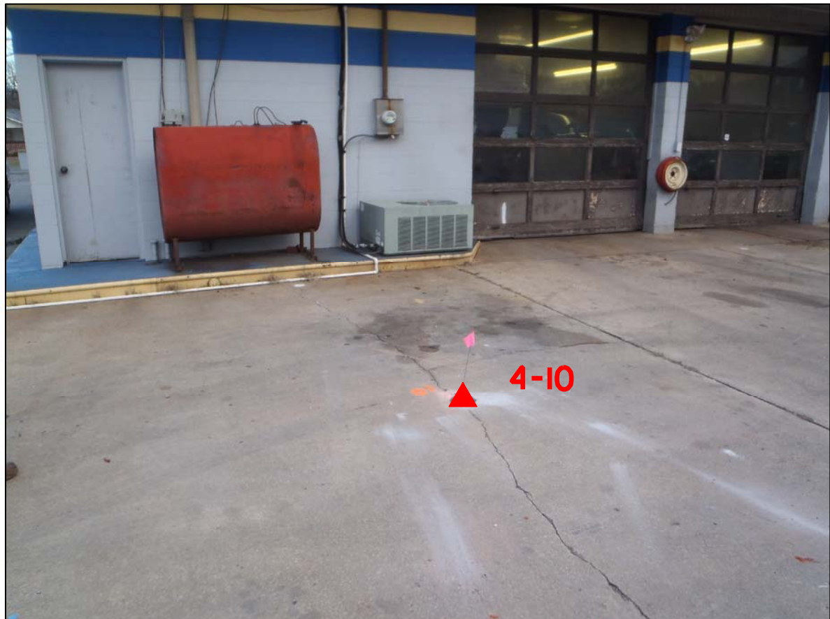
PHOTO 10 - BORING AT FUEL OIL AST LOOKING EAST
