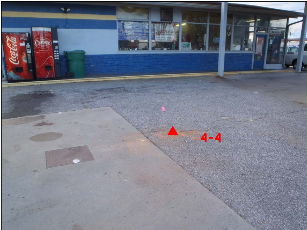
PHOTO 4 - BORING AT EXISTING UST BASIN LOOKING WEST
