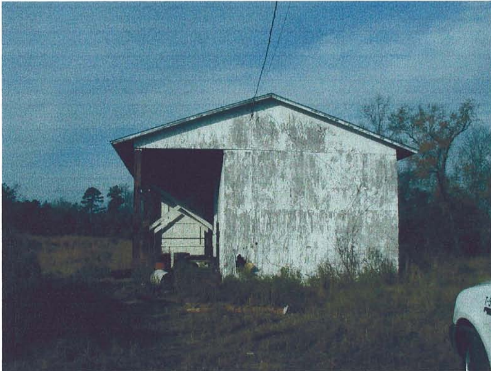
Photograph No. 5: Former garage where the equipment was serviced during the landfills operation.
