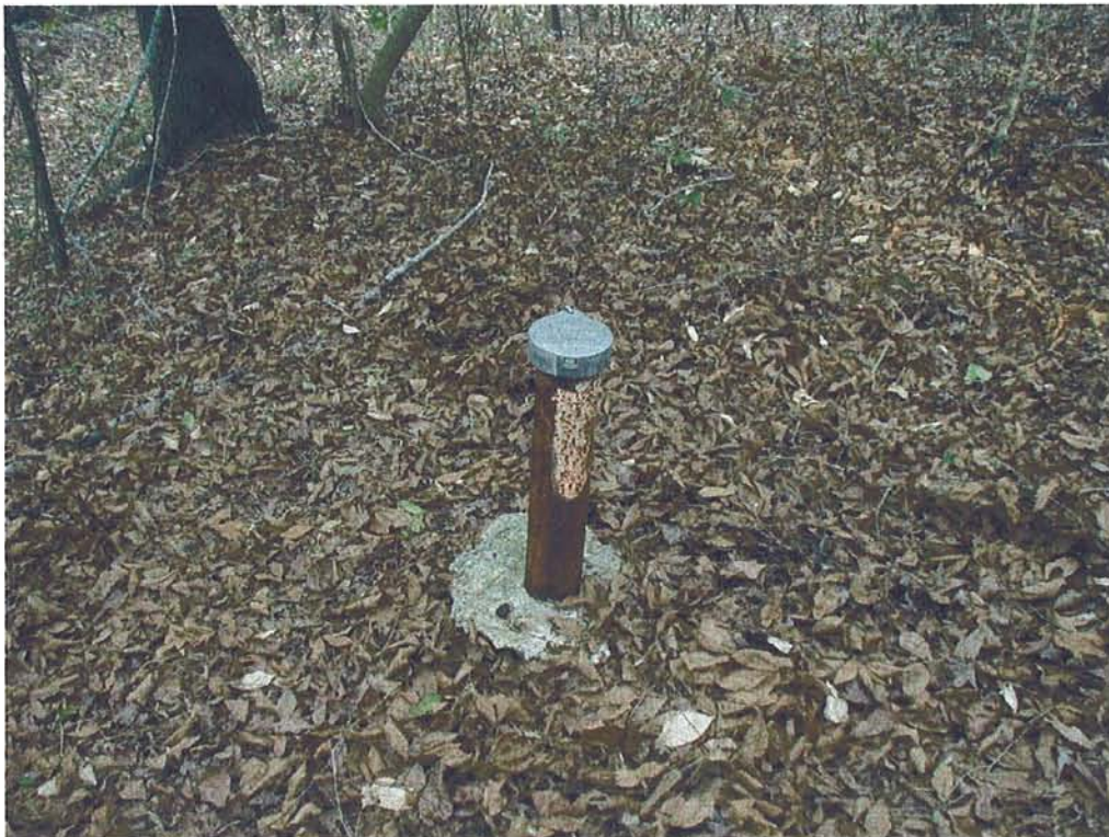
Photograph No. 8: One of nine monitoring wells that were installed along the perimeter of the site.
