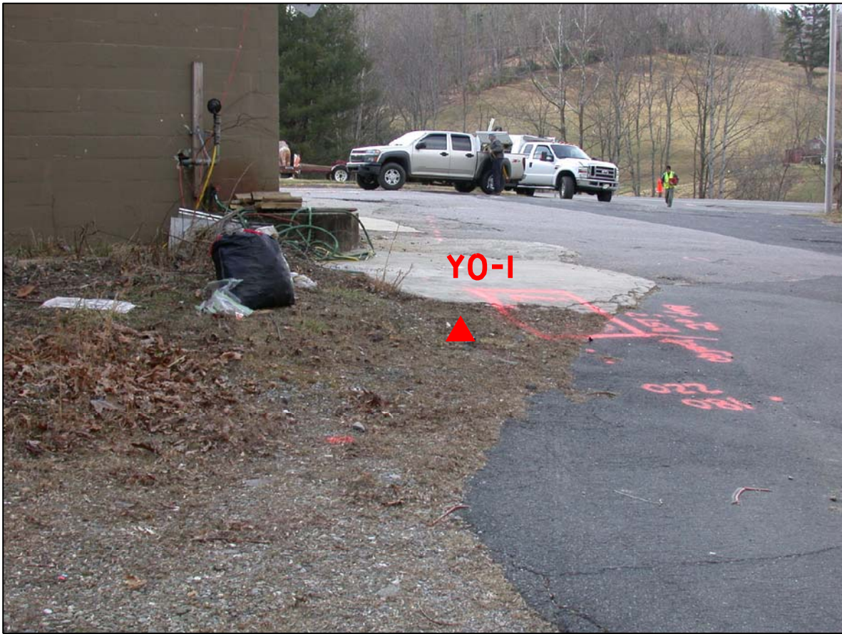
PHOTO 1 - BORING ON NORTH SIDE OF BUILDING AT ANOMALY LOOKING SOUTH
