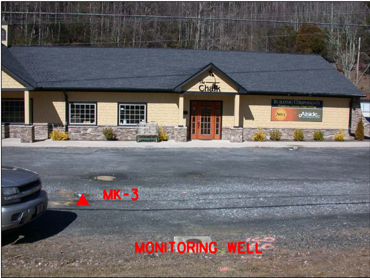
PHOTO 3 - BORING WITHIN RIGHT-OF-WAY LOOKING NORTH
