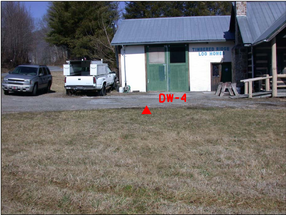
PHOTO 3 - BORING ON SOUTH SIDE OF BUILDING LOOKING NORTH
