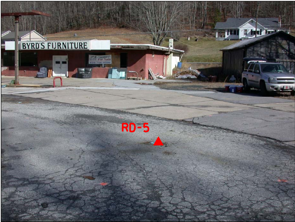
PHOTO 5 - BORING WITHIN RIGHT-OF-WAY LOOKING NORTHWEST
