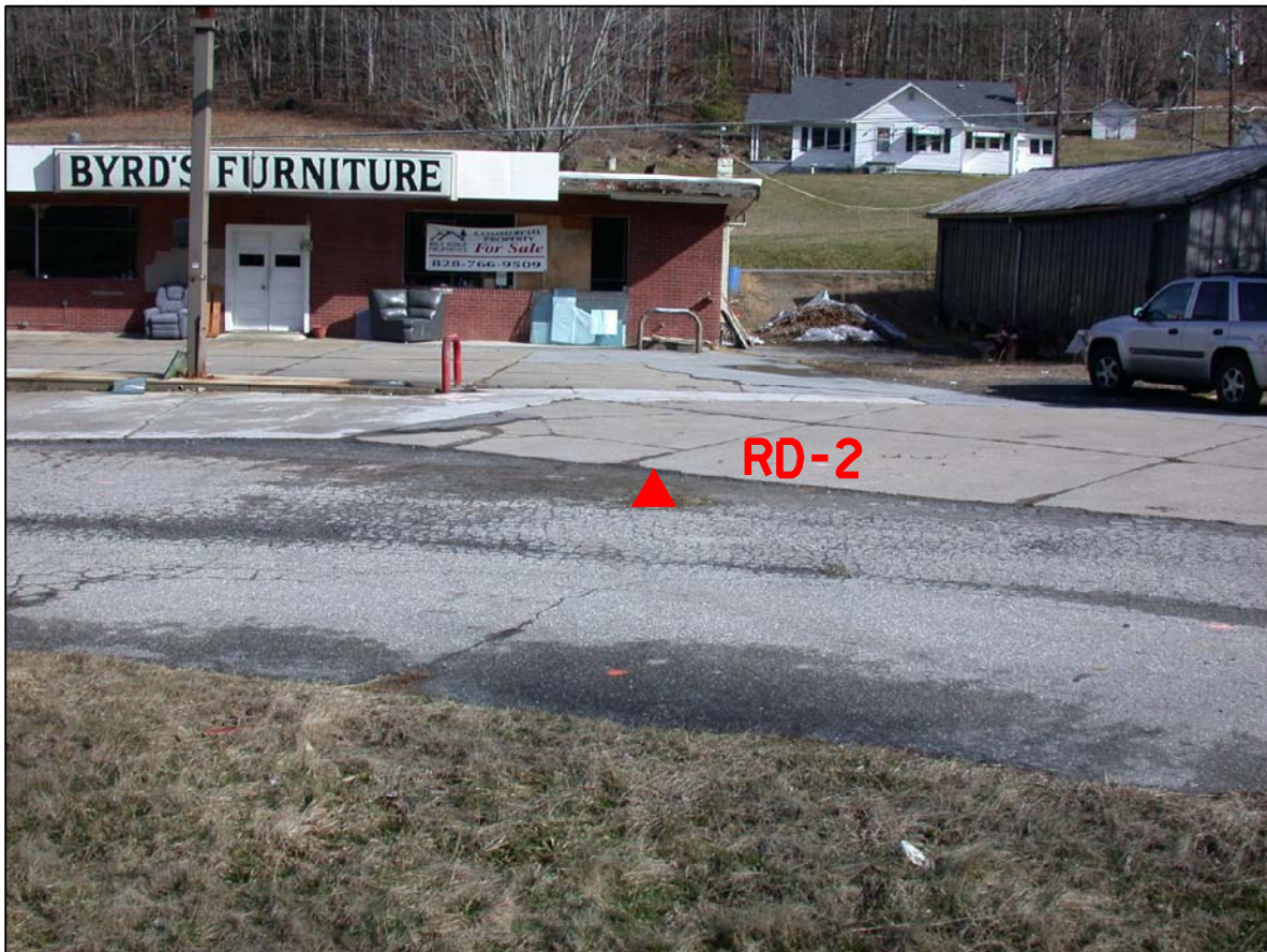
PHOTO 2 - BORING WITHIN RIGHT-OF-WAY LOOKING NORTH
