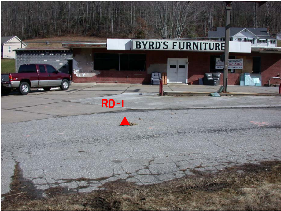
PHOTO 1 - BORING WITHIN RIGHT-OF-WAY LOOKING NORTH
