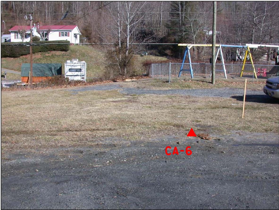
PHOTO 5 - BORING WITHIN RIGHT-OF-WAY LOOKING NORTH
