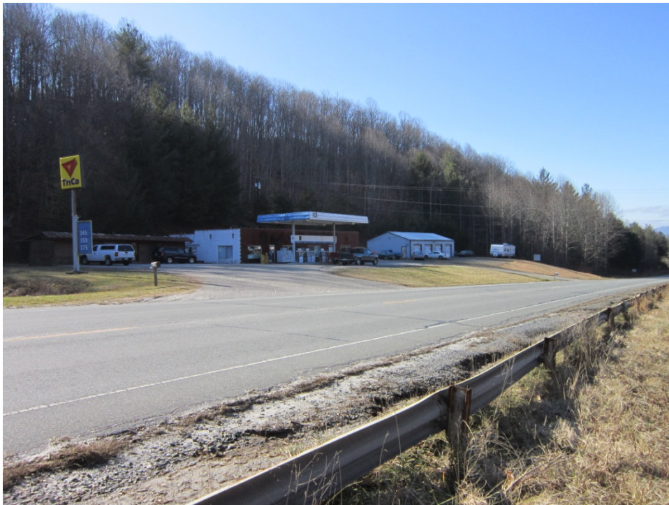
Parcel 76 (Tony and Veneta Honeycutt Property), looking southwest
