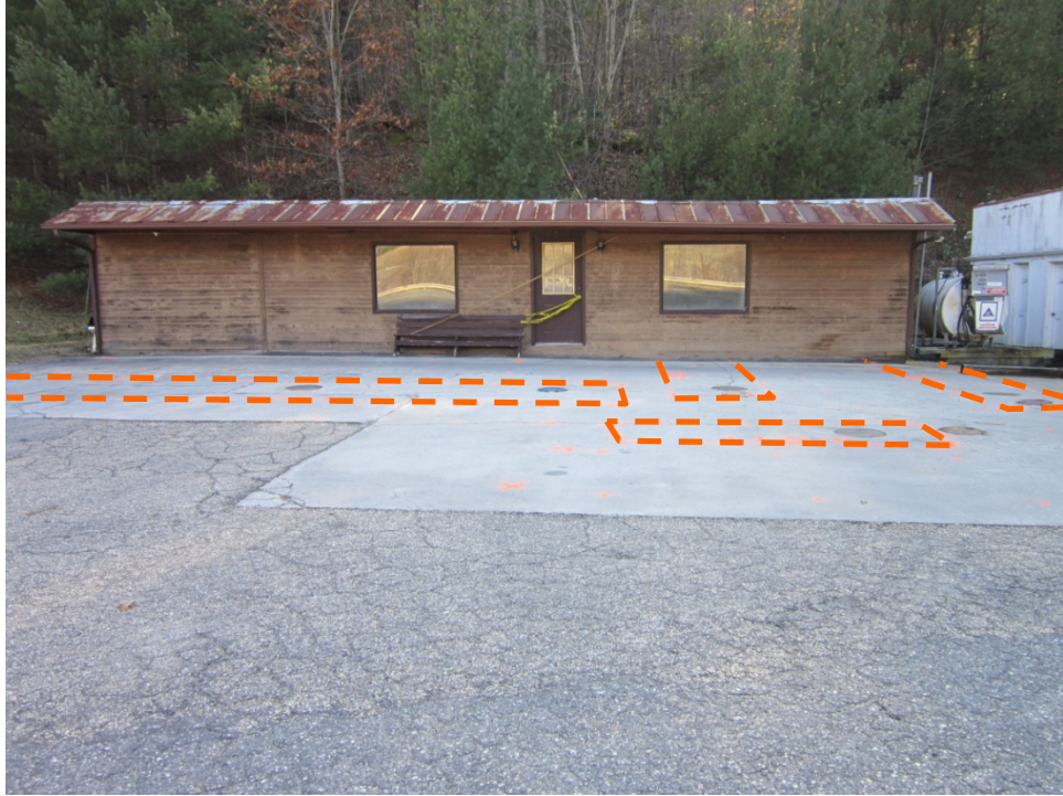
Parcel 76 (Tony and Veneta Honeycutt Property), looking south. Photo shows approximate marked locations of known UST Nos. 1 through 4 near the vacant building on the eastern side of the site.
