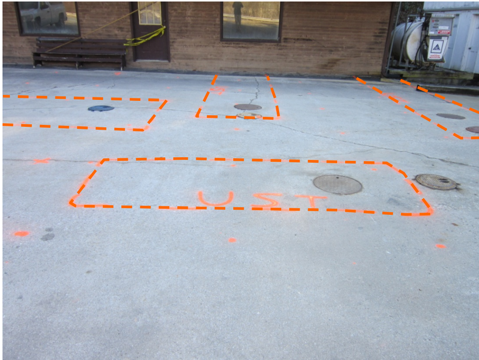
Parcel 76 (Tony and Veneta Honeycutt Property), looking southwest. Photo shows approximate marked locations of known UST Nos. 1 through 4 near the vacant building on the eastern side of the site.
