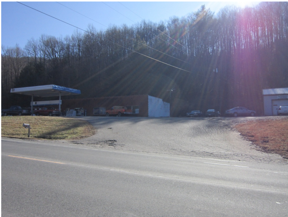
Parcel 76 (Tony and Veneta Honeycutt Property), looking south
