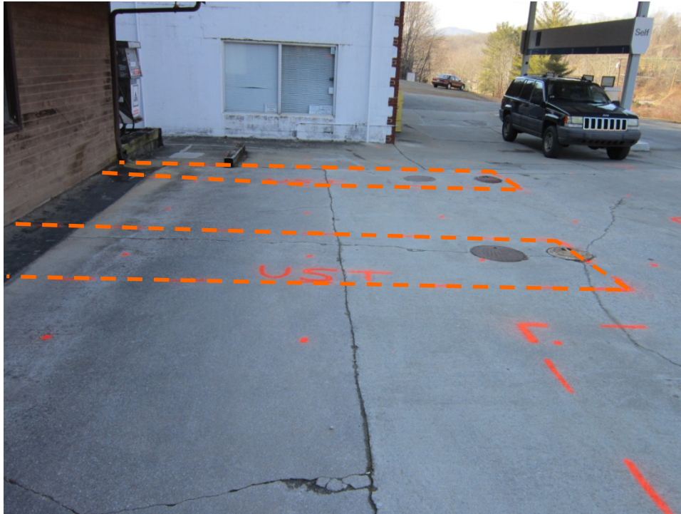
Parcel 76 (Tony and Veneta Honeycutt Property), looking northwest. Photo shows approximate marked locations of known UST Nos. 1 and 2 near the vacant building on the eastern side of the site.
