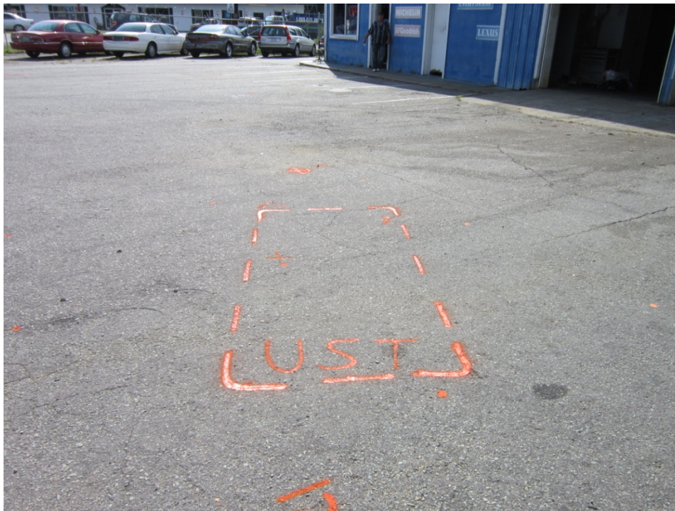
Parcel 202 (Tsoumbos Aristotelis Property), looking west. Photo shows approximate marked location of Possible UST No. 1 near the south side of the building.
