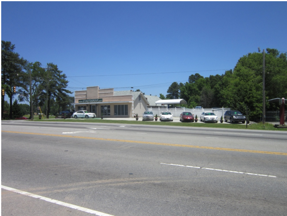
Parcel 189 (Northern Holdings LLC Property), looking northeast
