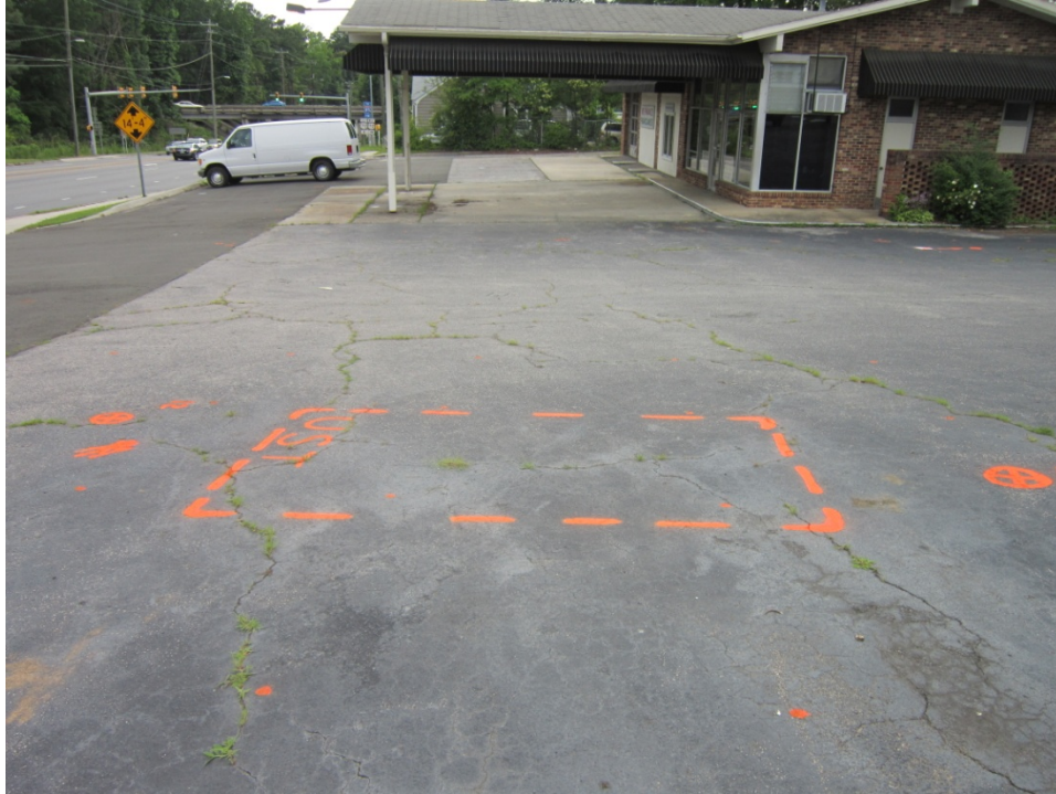
Parcel 128 (William E. Andrews Property), looking west. Photo shows approximate marked location of Probable UST No. 1 near the southeast corner of the parcel.
