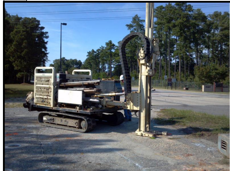
8 Advancing boring B-4 after drill rods were exchanged.
