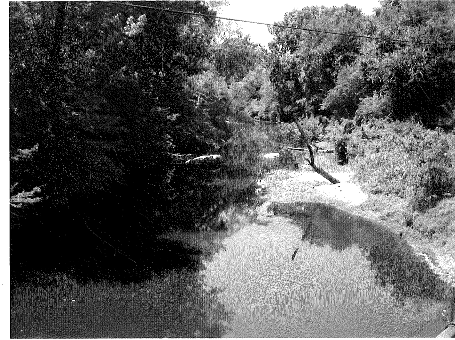
Photograph No. 11: This photograph was taken from the right side of the -L- alignment, from the existing bridge deck, looking southeast (downstream).
