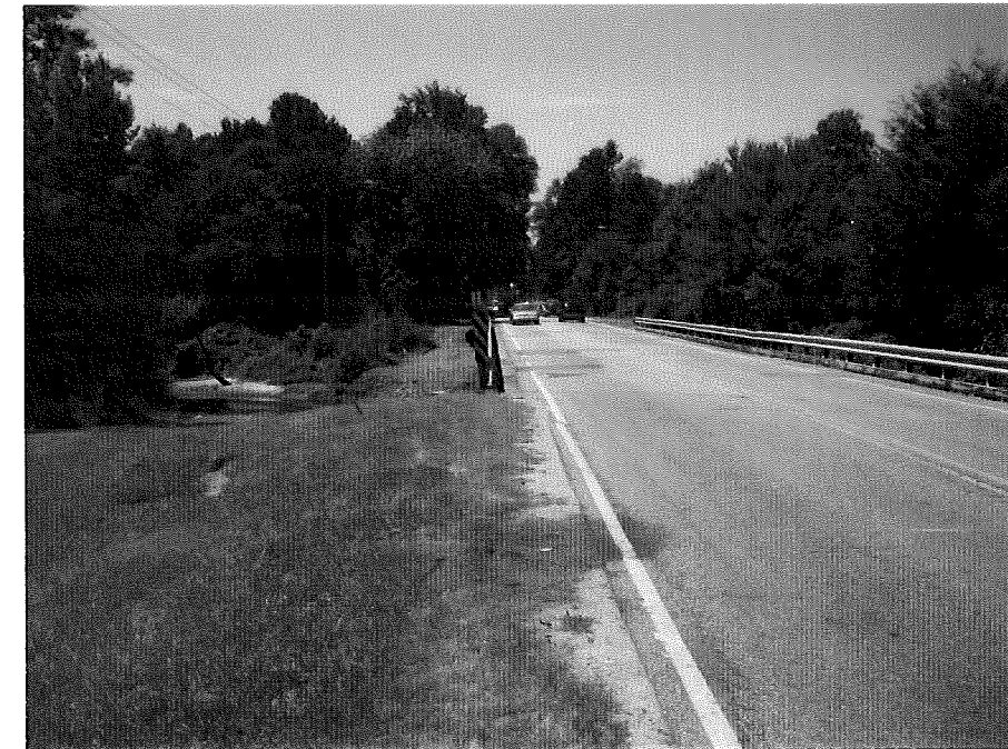
Photograph No. 16: This photograph was taken from the north approach, along the -L- alignment, looking southwest.
