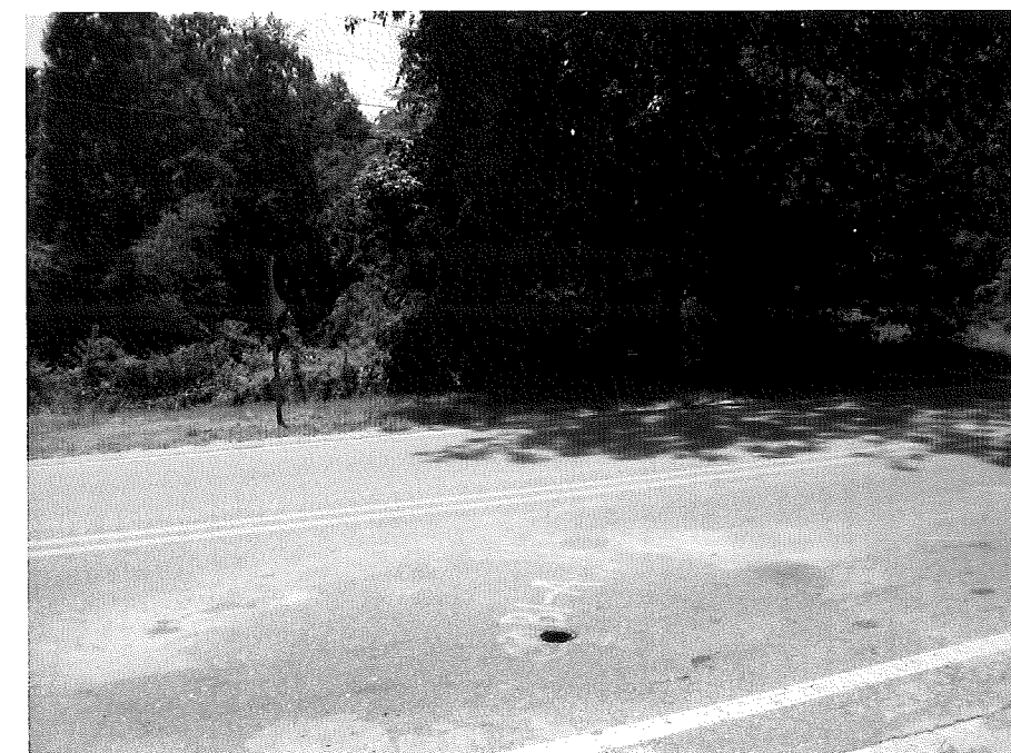
Photograph No. 4: This photograph was taken from the left side of the -L- alignment, looking southeast, across proposed Interior Bent No. 1.
