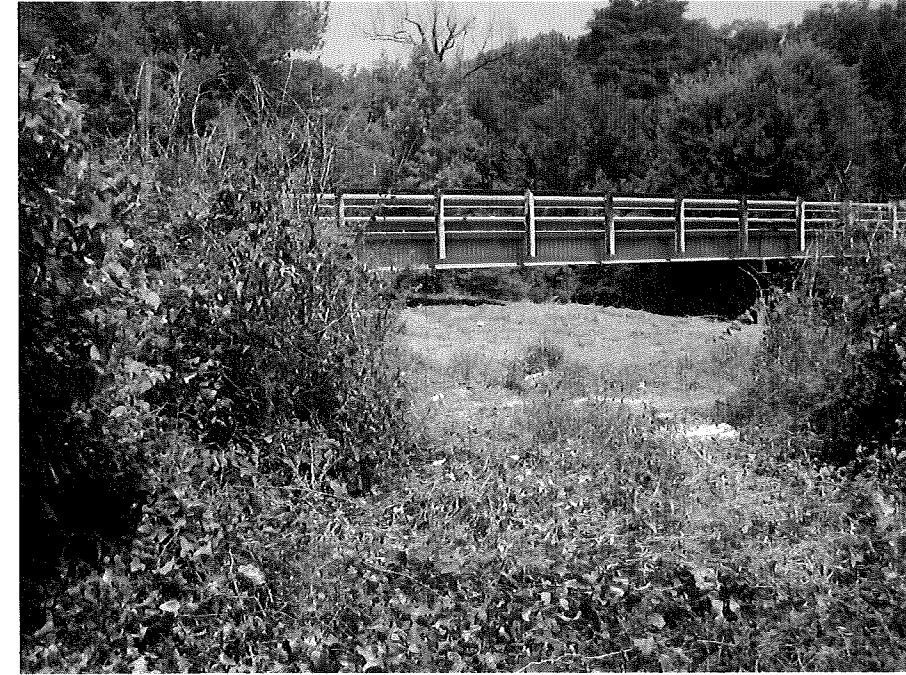
Photograph No. 7: This photograph was taken from the right side of the -L- alignment, looking northwest, across proposed Interior Bent No. 2.
