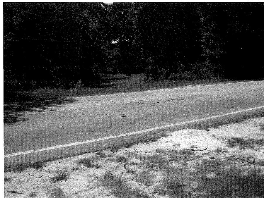
Photograph No. 2: This photograph was taken from the left side of the -L- alignment, looking southeast, across proposed End Bent No. 1.
