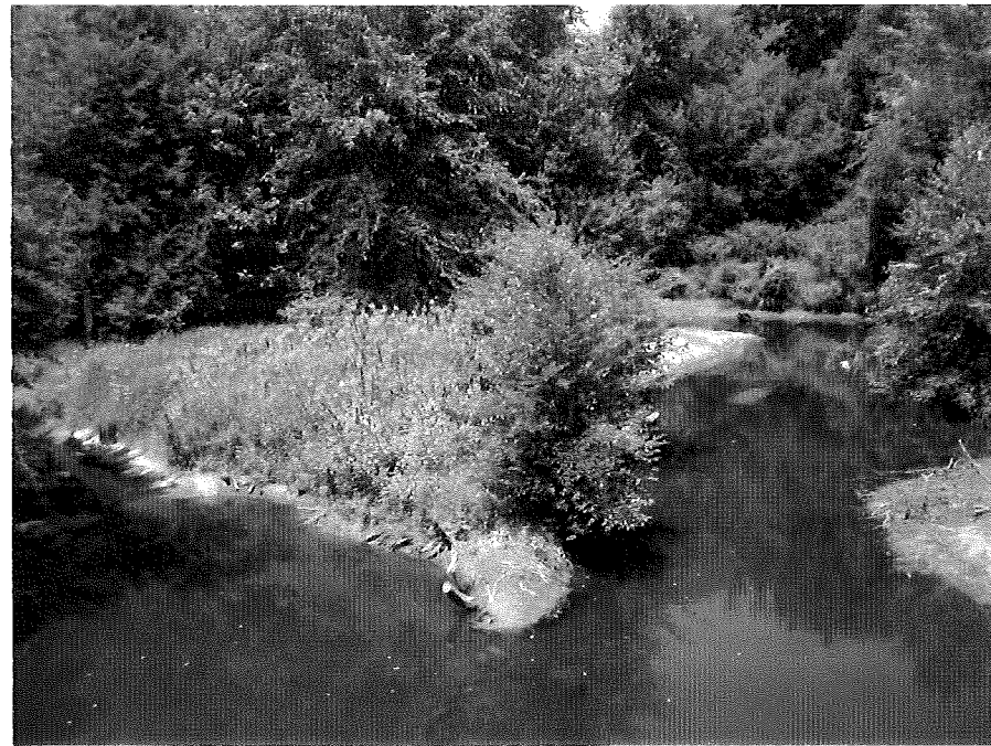
Photograph No. 10: This photograph was taken from the left side of the -L- alignment, from the existing bridge deck, looking northwest (upstream).
