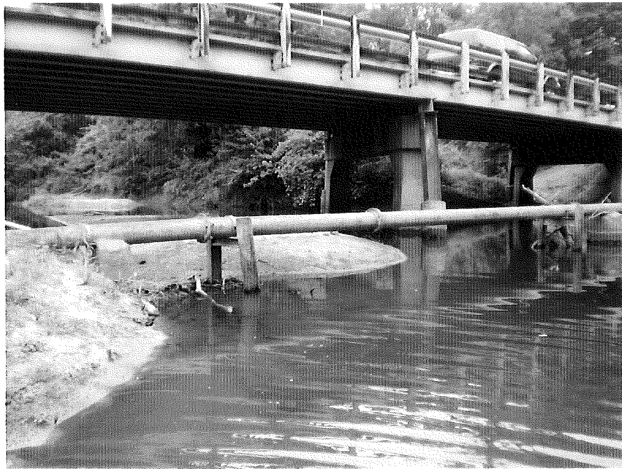
Photograph No. 9: This photograph was taken from the right side of the -L- alignment, looking northwest, across proposed Interior Bent No. 3.
