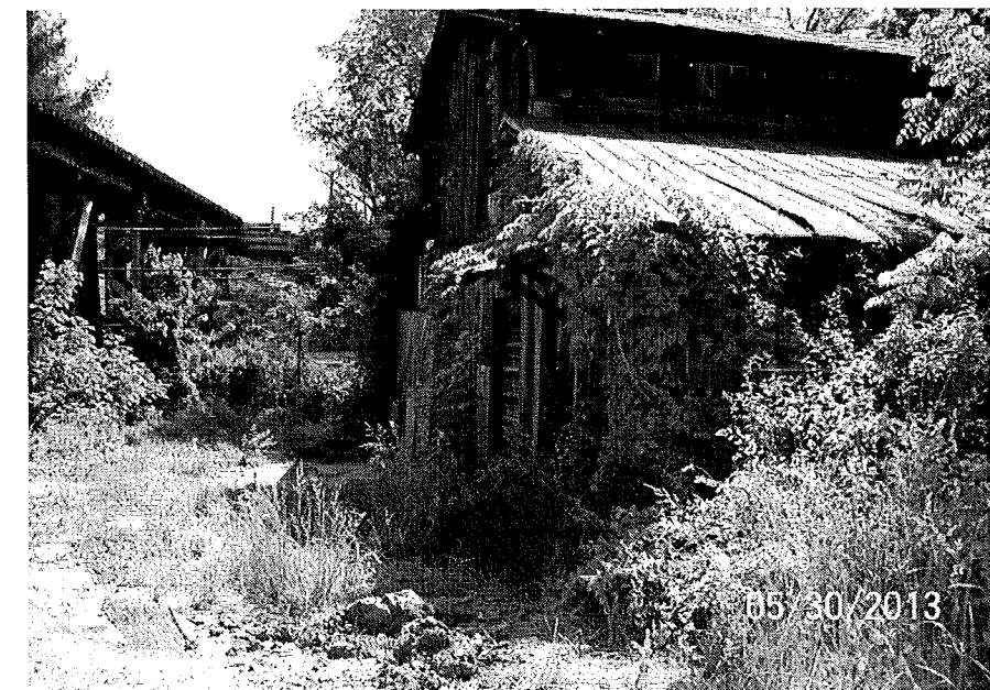
View Looking Downstation From End Bent-2
