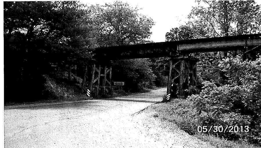
View of Existing Bridge Looking South
