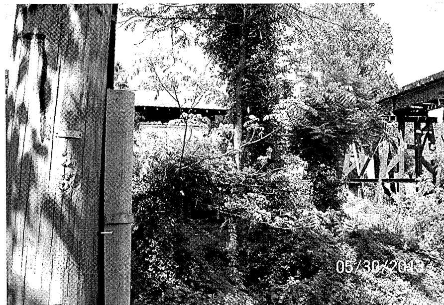
View Along CL Looking Upstation from NC 209
