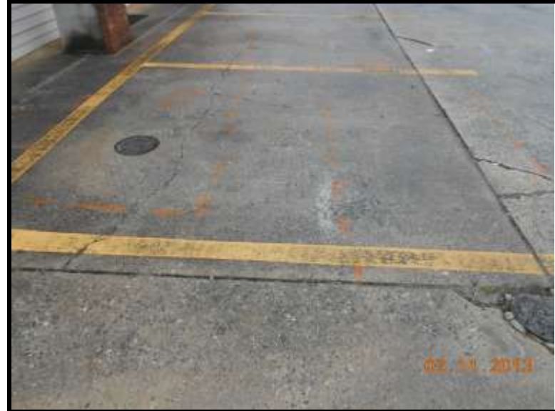
2 View of Anomaly 1 with probable UST's outlined with orange spray paint. View is to the northeast.
