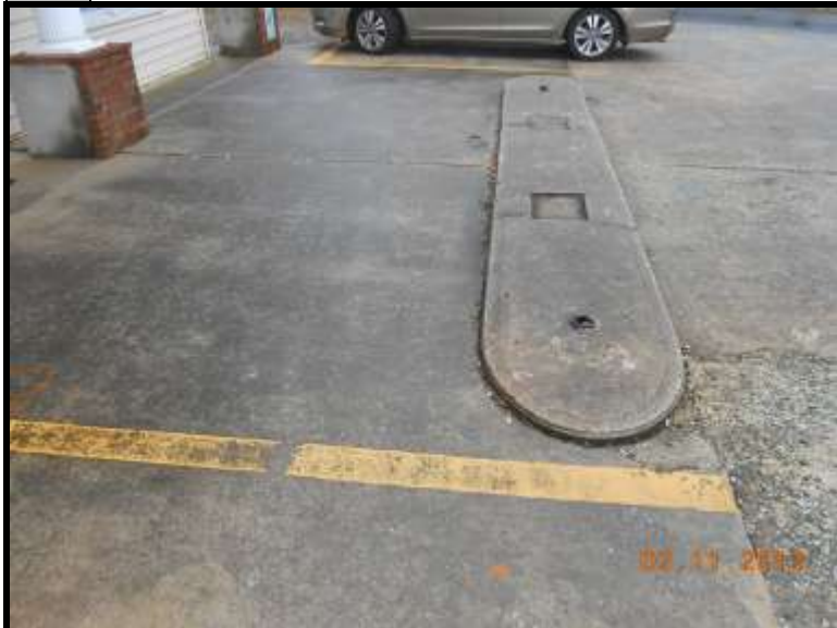
3 View of former dispenser island in parking lot of A Step Above Denture Services. View is to the northeast.
