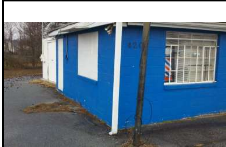
2 View of the southwestern corner of Cutterz Barbershop facing northeast.
