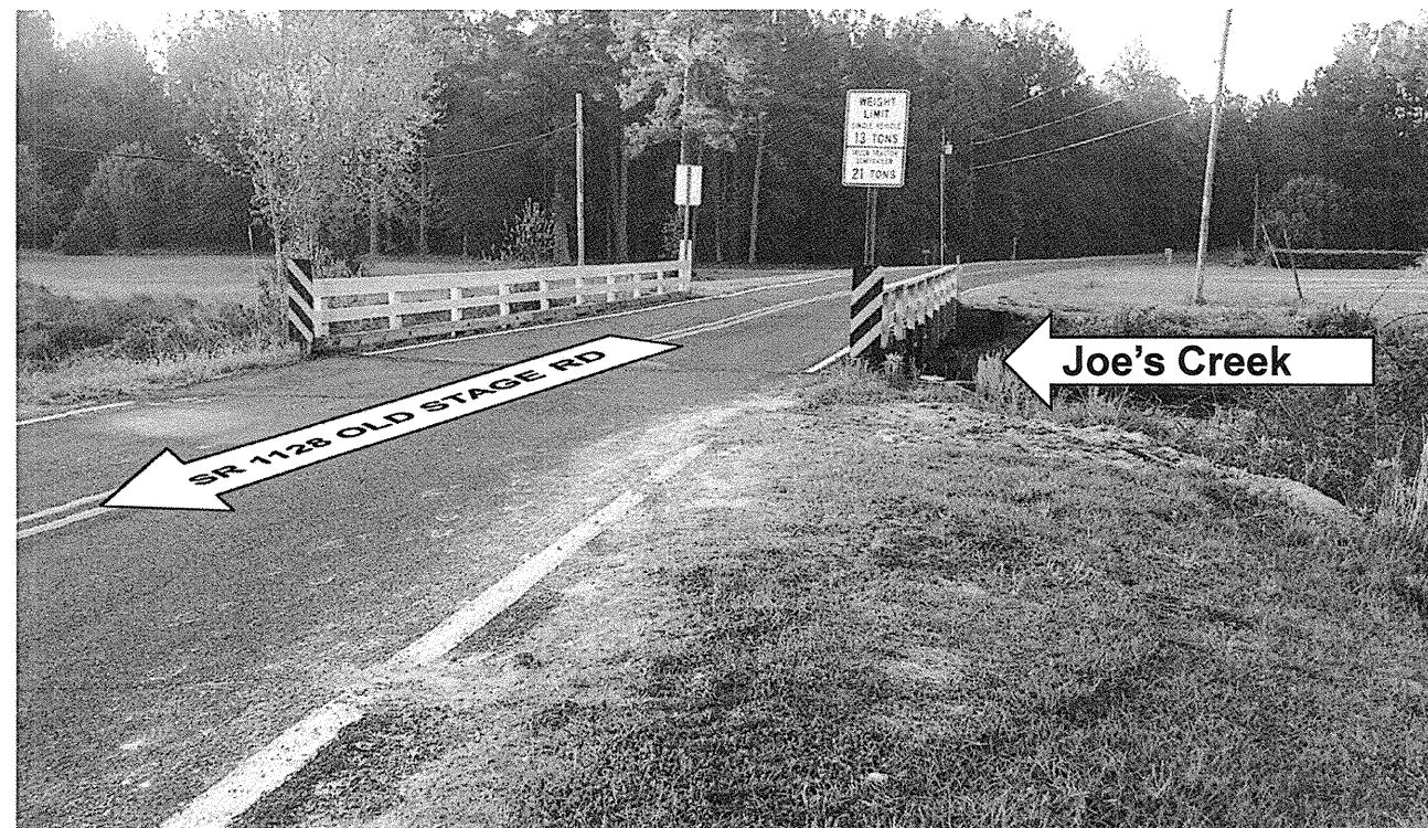
Bridge No. 63 – Looking South
