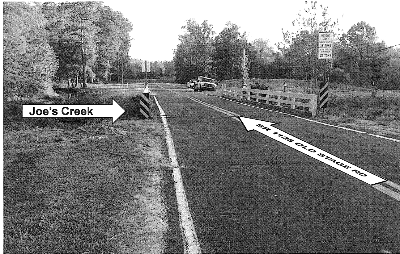
Bridge No. 63 – Looking North
