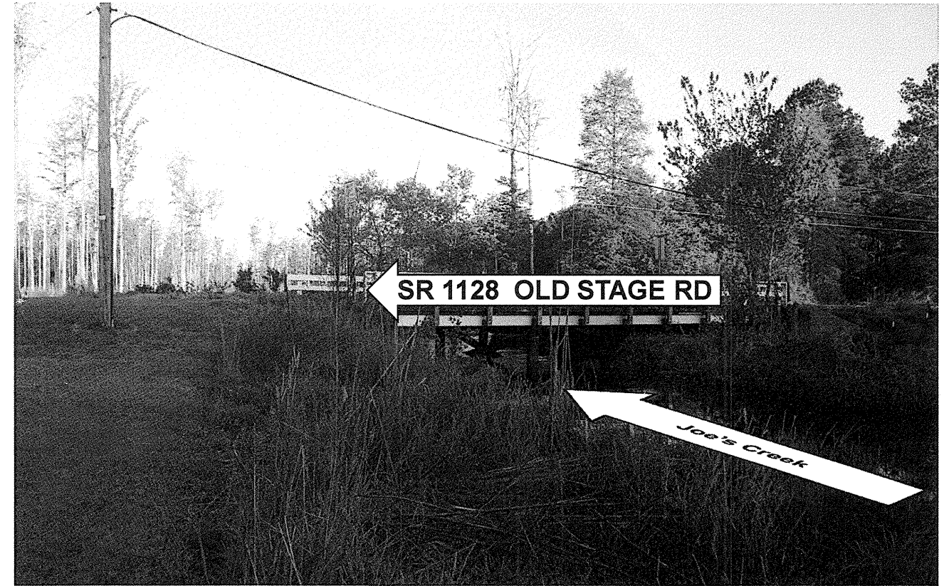
Bridge No. 63 – Looking East
