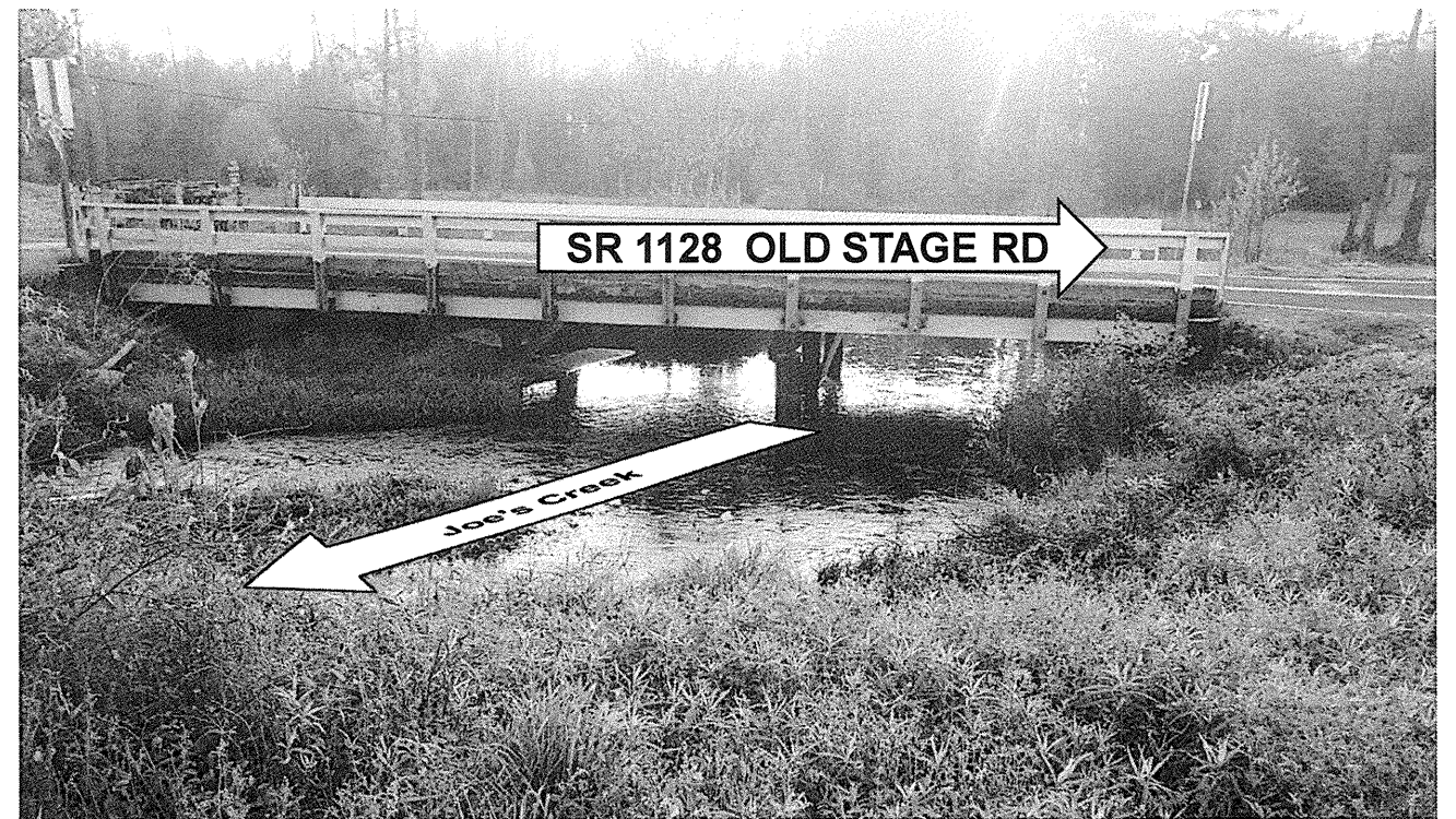
Bridge No. 63 - Looking West
