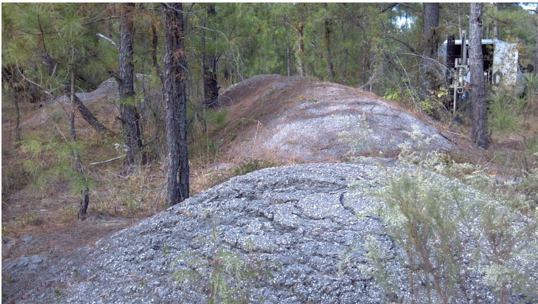
Photo #8: View of asphalt stockpiles in the vicinity of Borings B-15 and B-16
