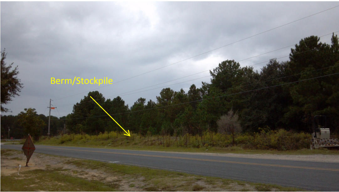
Photo #3: Frontage of site along the east side of Sandy Ridge Church Road. The berm/stockpile shown consists of crushed asphalt for the entire length of roadway from the site entrance to US 220.
