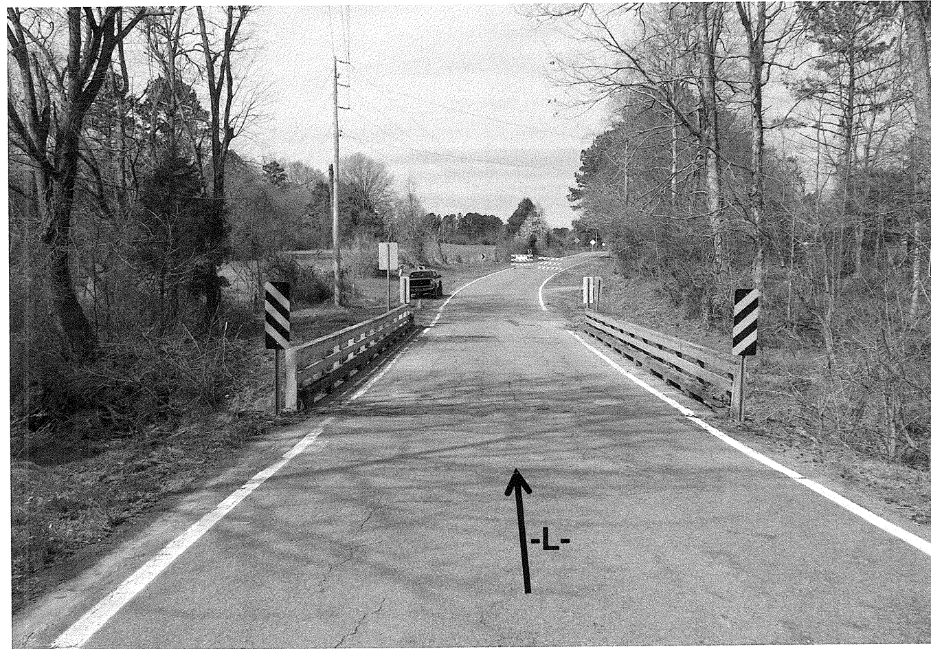
View of SR 2159 looking West
