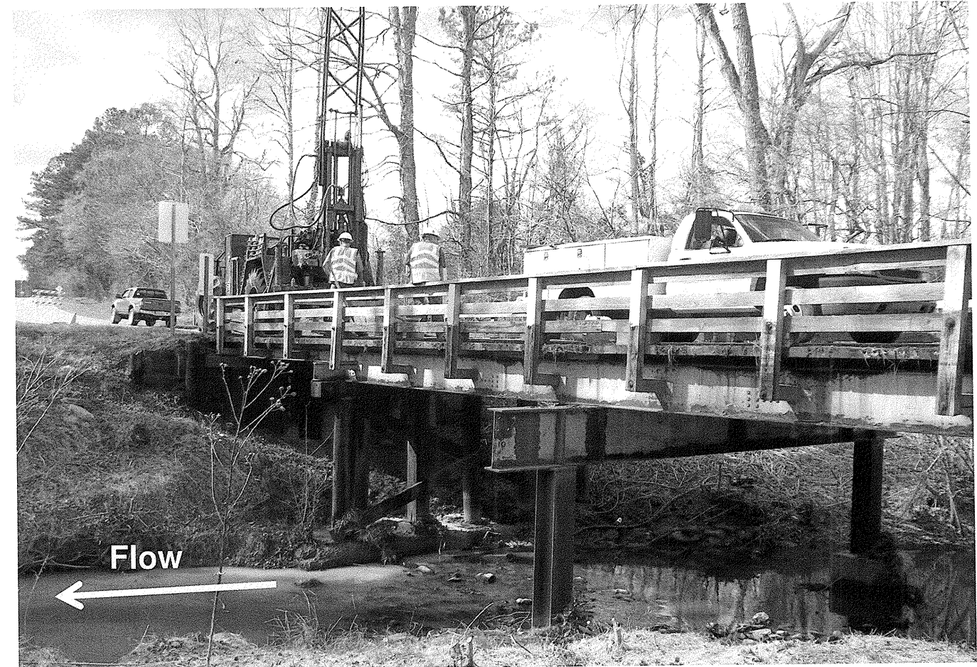
View of Bridge No. 129 looking Northwest
