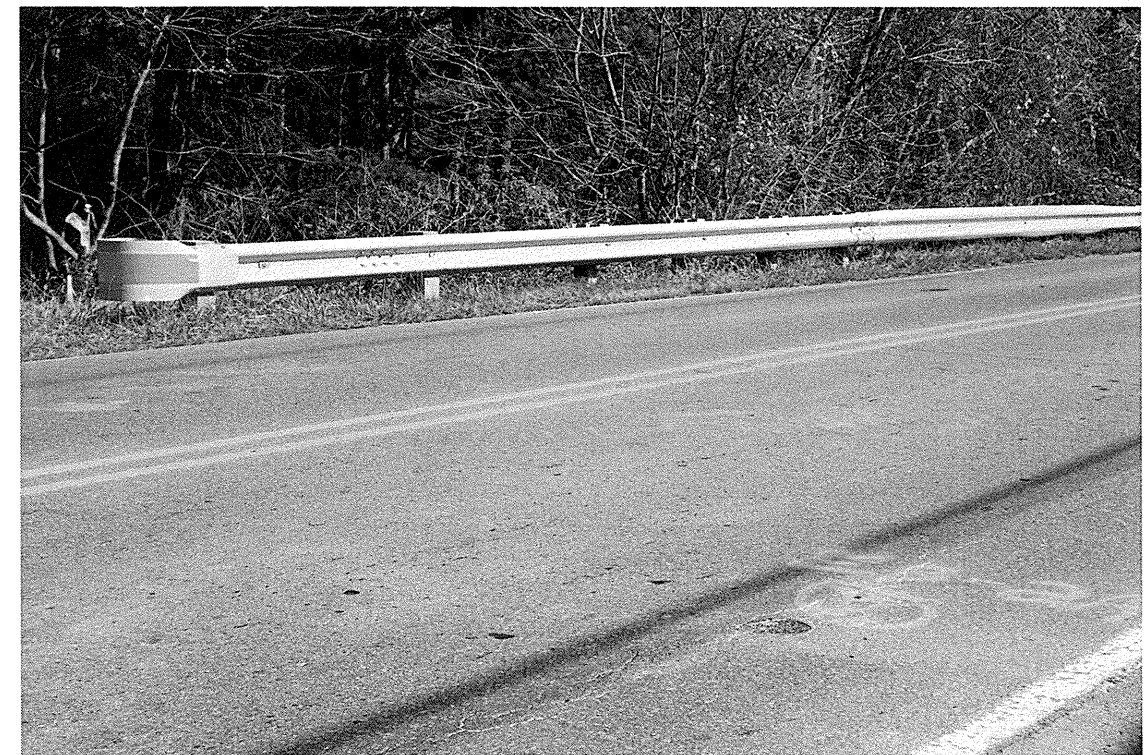
End Bent 2: Looking left to right.
