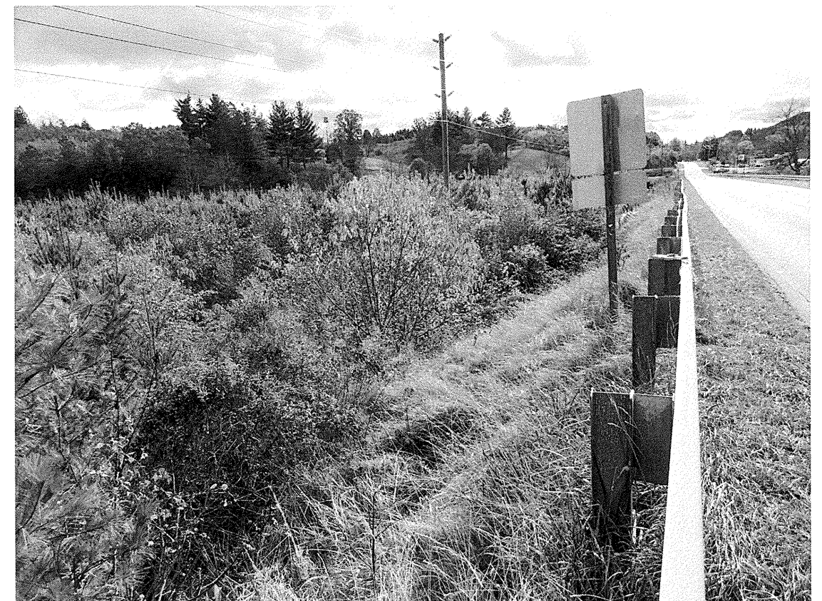
Looking down station right of -L-
