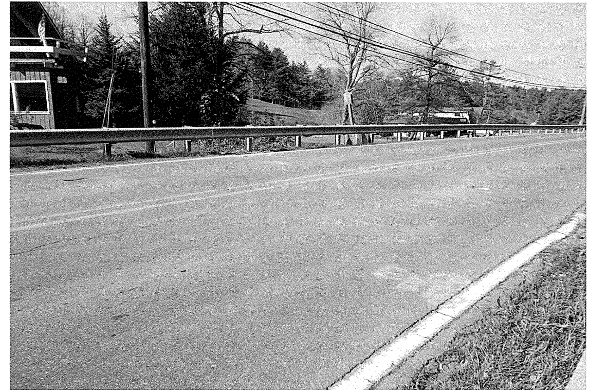
End Bent 1: Looking right to left.
