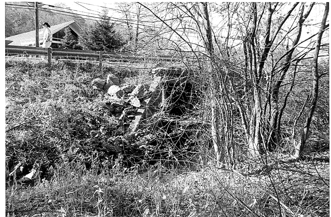
Looking down stream at existing culvert
