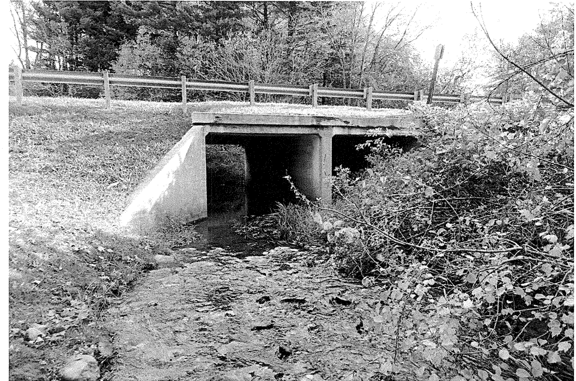
Looking up stream at existing culvert
