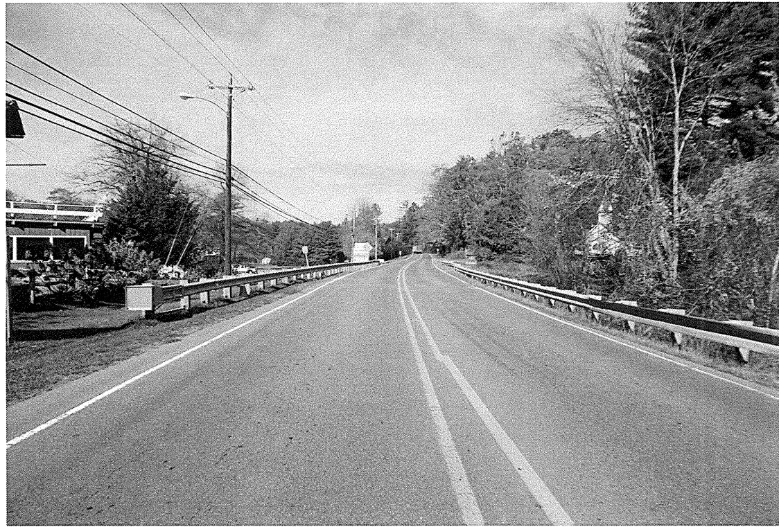
Looking up station at site
