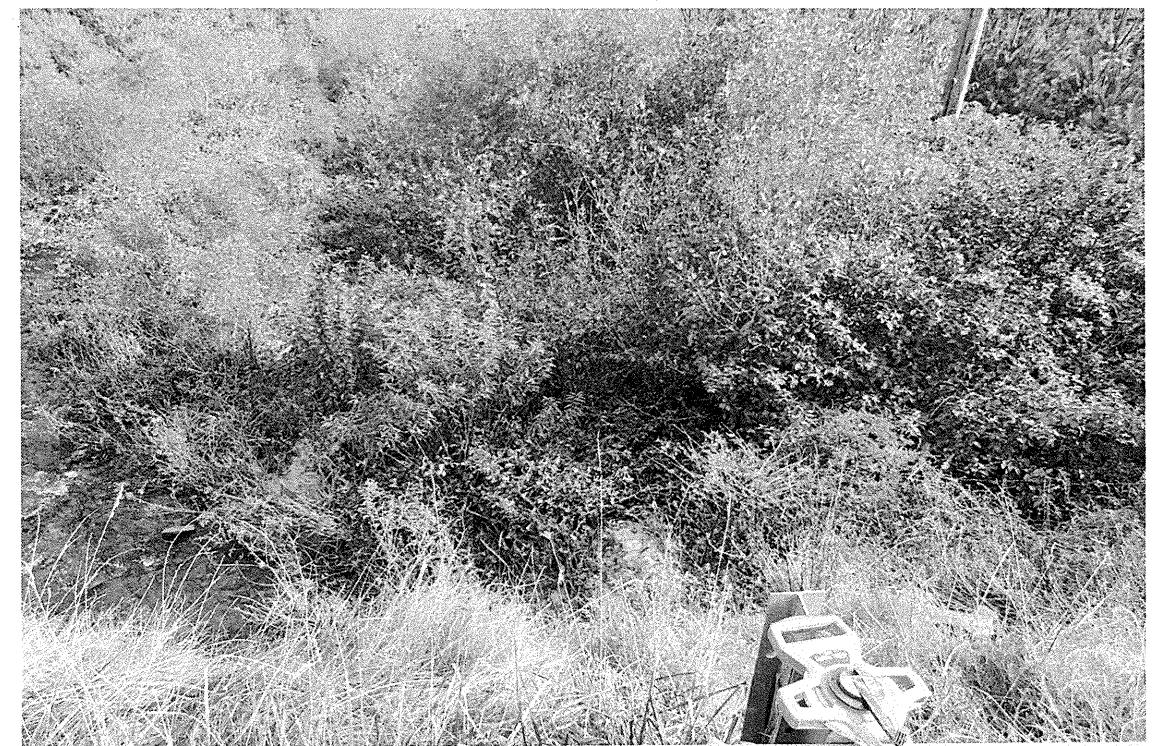
Looking down the embankment right of -L- from road side at B1
