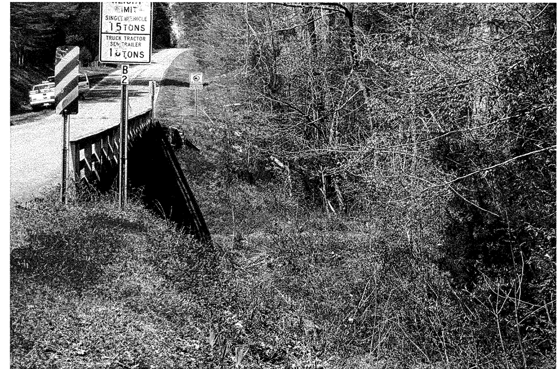
Looking down station left of -L- from End Bent 2
