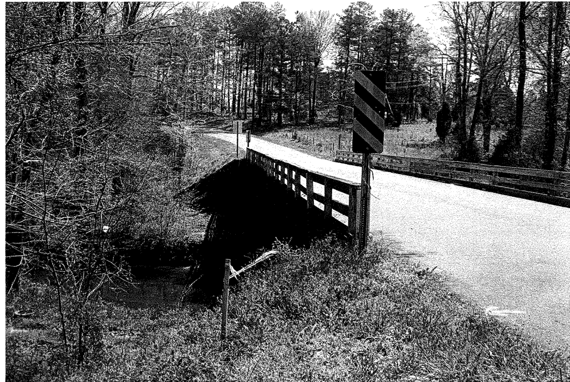
Looking up station left of -L- from End Bent 1
