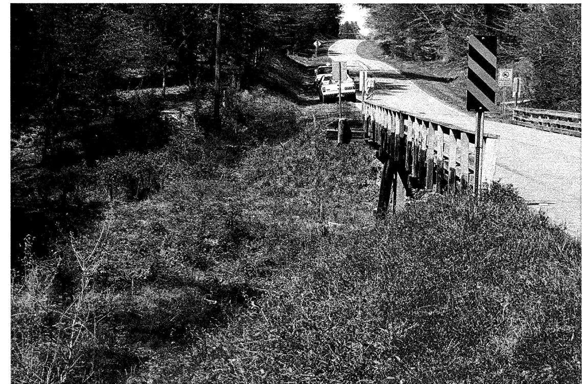
Looking down station right of -L- from End Bent 2
