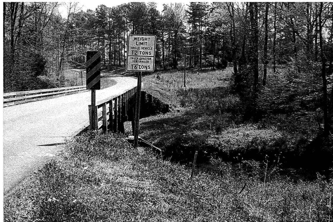
Looking up station right of -L- from End Bent 1
