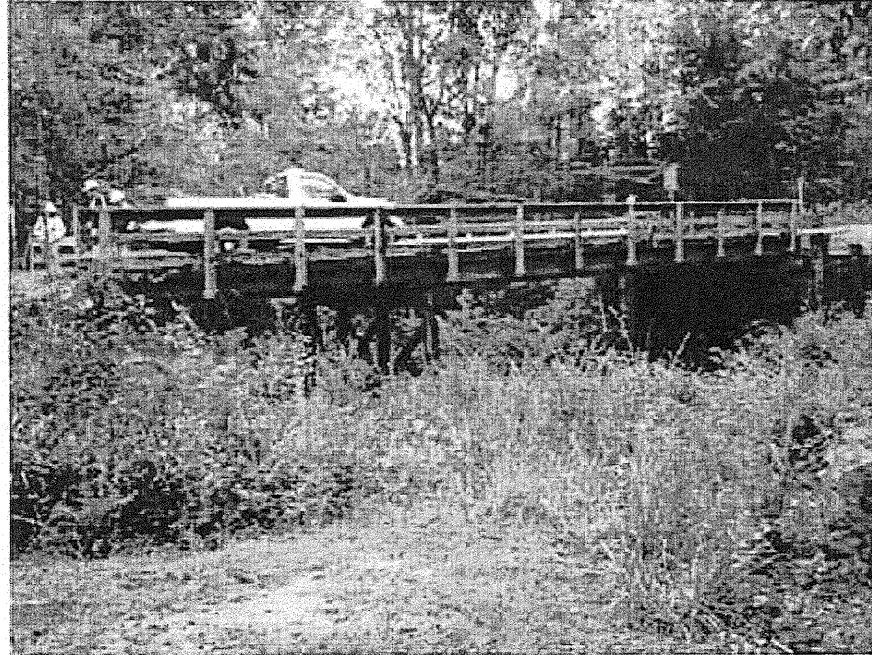
Photograph No. 1: General view of the bridge site looking west
