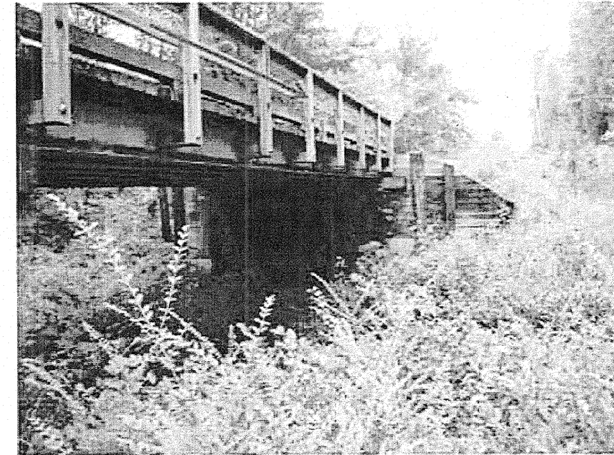
Photograph No. 4: View looking north towards existing End Bent 2
