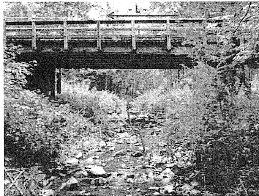
Photograph No. 2: View looking upstream towards End Bent 2 & Bent 1
