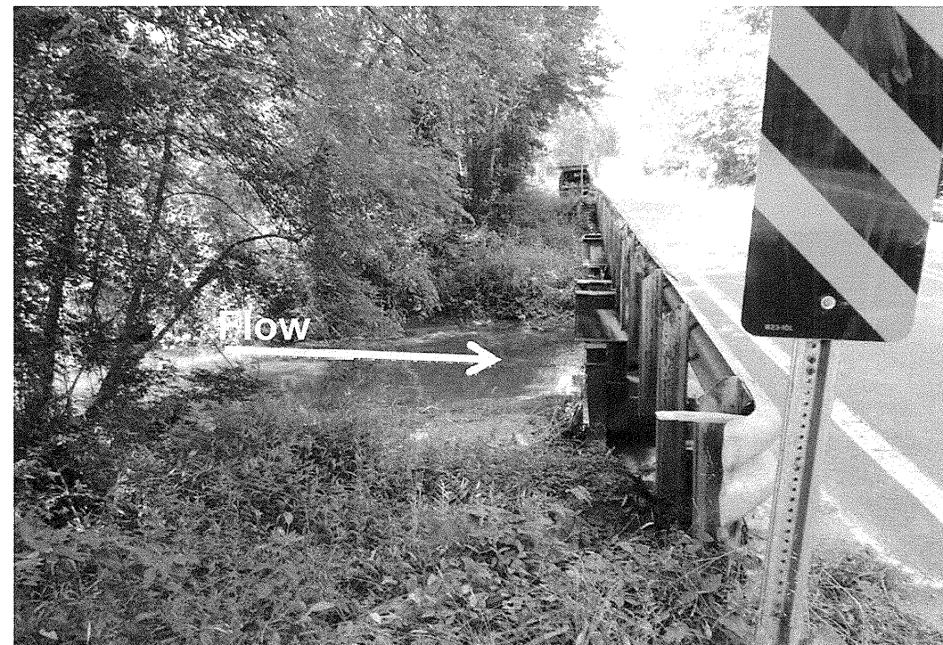
View of Northwest side of Bridge No. 120 looking Northeast
