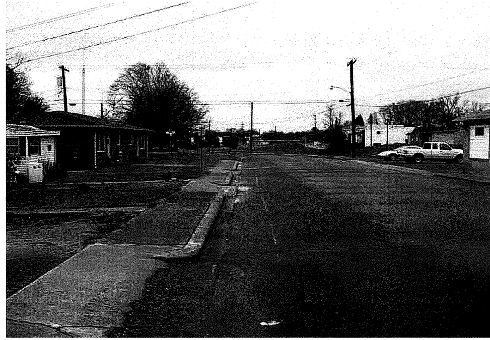
View Looking Upsation along Retaining Wall A alignment from Station 13+00
