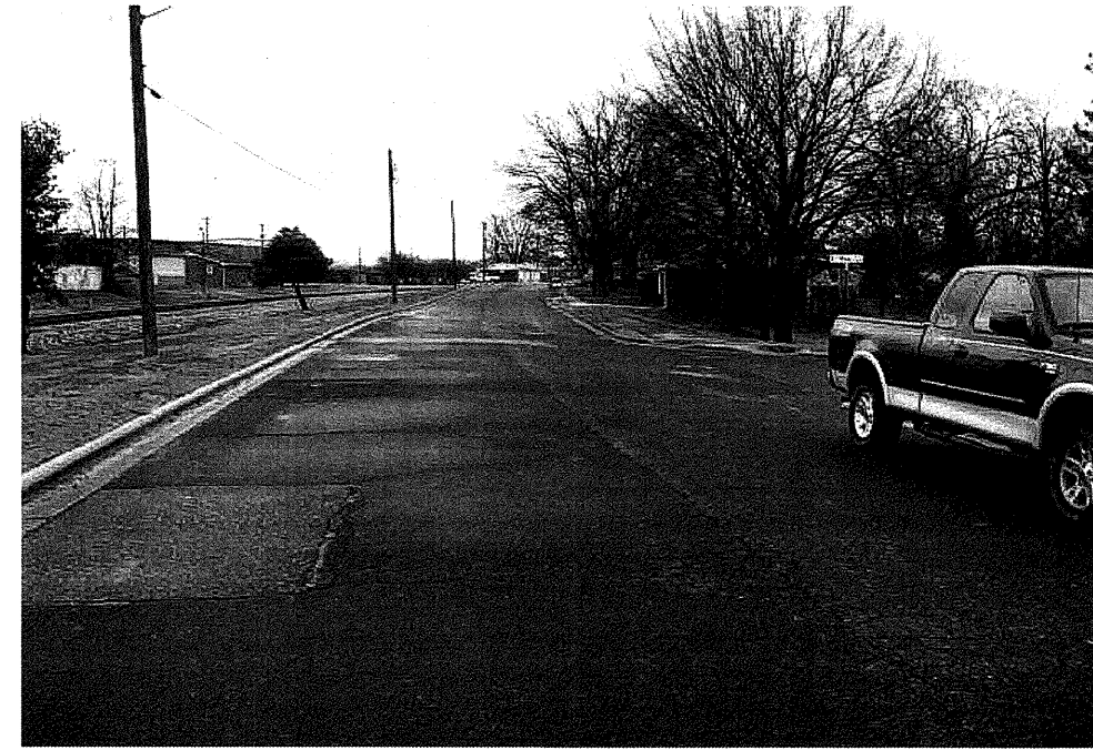
View Looking Downstation along Retaining Wall A alignment from Station 19+81
