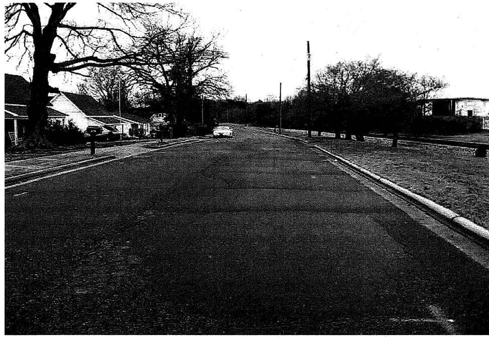
View Looking Upsation along Retaining Wall A alignment from Station 19+81
