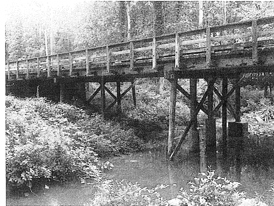
Photograph No. 3: View looking downstream towards existing Bents 1 and 2
