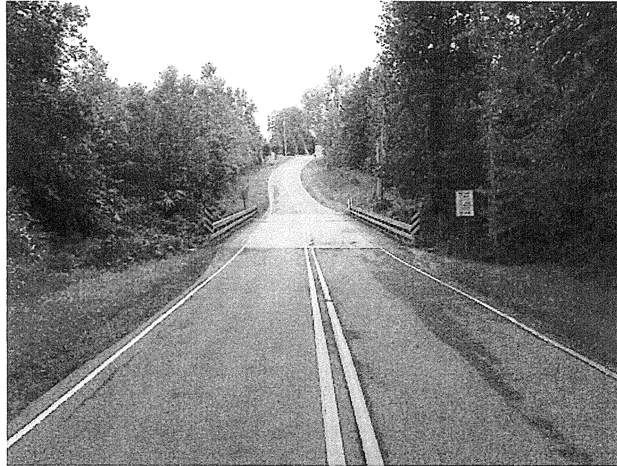
Photograph No. 1: General view of the bridge site looking north
