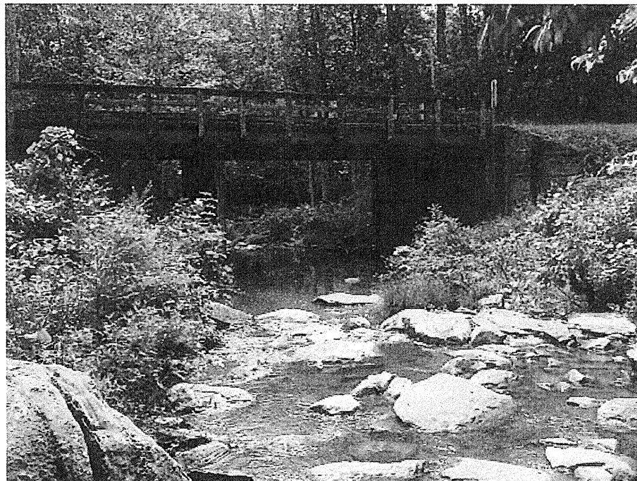
Photograph No. 2: View looking downstream towards existing End Bent 1
